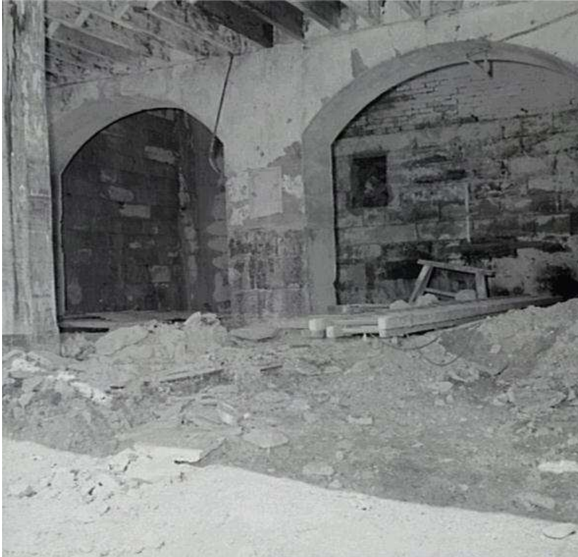
Figure 2: Photograph of sandstone vaulted archways under Macquarie Street, 1964 appears to show demolition in process. (Source: City of Sydney Archives, Citation: NSCA CRS 48/3825).
