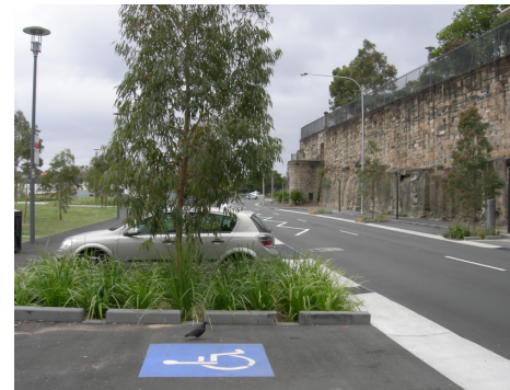
Street tree bioretention systems to treat runoff from Porter Street equating to approx. 30m 2 of bioretention area to be provided. The final number of trees will be dependant on available space and position of existing trees.
