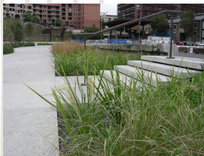
A linear bioretention system with a 320m 2 footprint will treat runoff from southern catchment.
