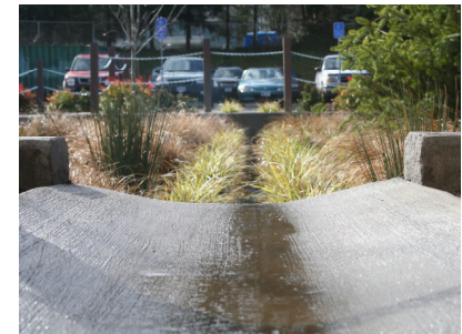
Stormwater treatment wetland and water body with a 150m 2 footprint. The system treats all the surface runoff from the northern catchment including approx 5% of the roof area from blocks B, C and D. The remaining roof area drains to rainwater tanks and/or OSD.
