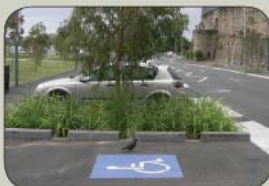
Street Tree Bioretention System
