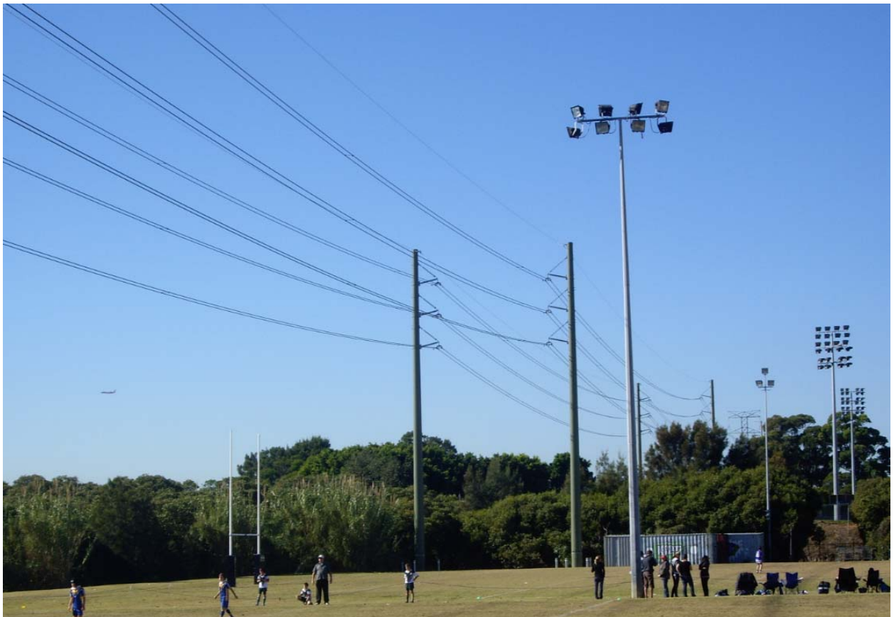
Photo #2 Two steel poles of 132kV Kurnell power line (feeder No:916 is suspended on the right and feeder No:917 is on the left poles ).
