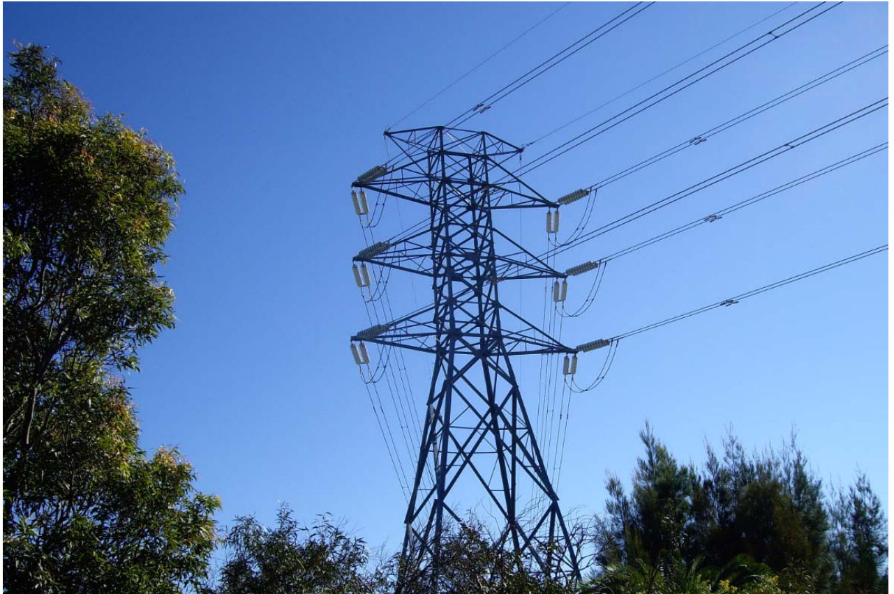
Photo #1 Steel tower of 132kV Kurnell power line (feeder No:916 is on the left and feeder No:917 is on the right )
