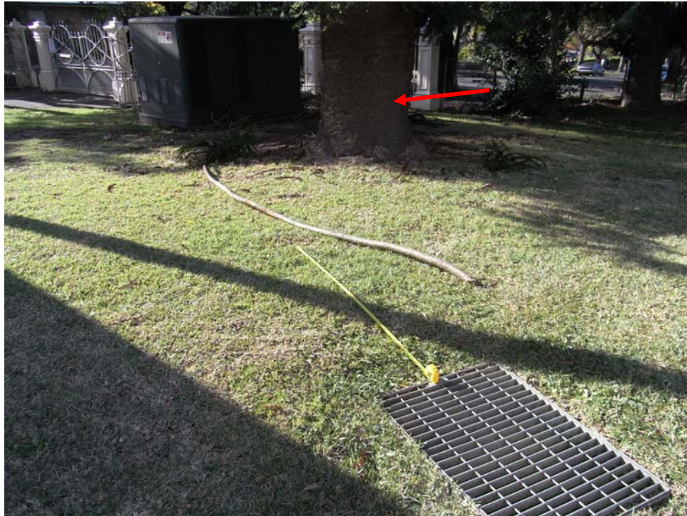
Photograph 3: Tree # 8 - Illustrating the electricity substation, Pit and stormwater pipe at 800mm depth and of ca. 300mm diameter in close proximity to tree (trunk arrowed) – the direction of the pipeline is depicted by tape measure - past damage to roots from installation of these facilities is not known to Landscape Matrix.
