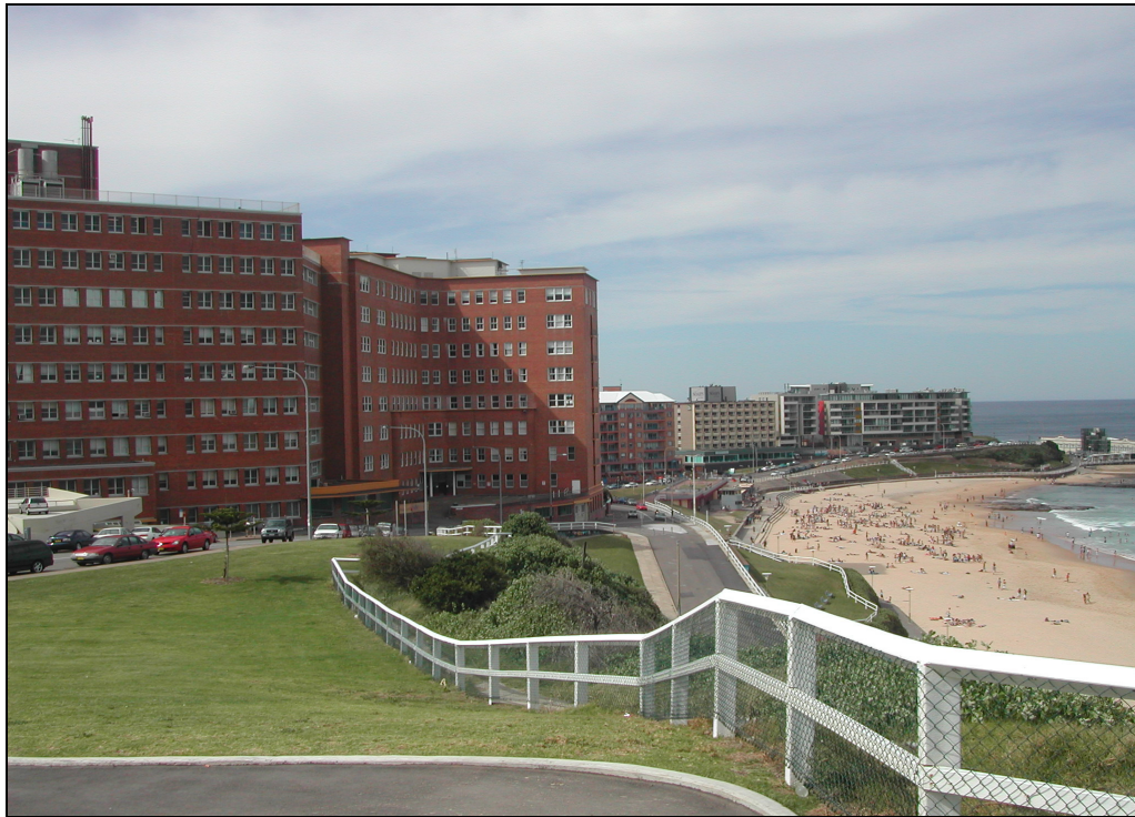
Photograph 1: Royal Newcastle Hospital looking north along Newcastle Beach
