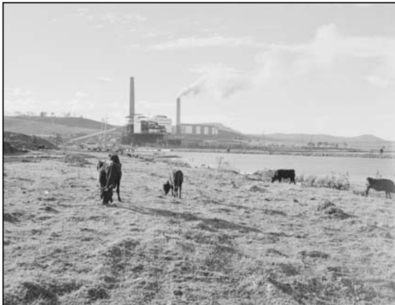
Figure 6: Tallawarra Power Station 1960 (Source: National Archives of Australia)
