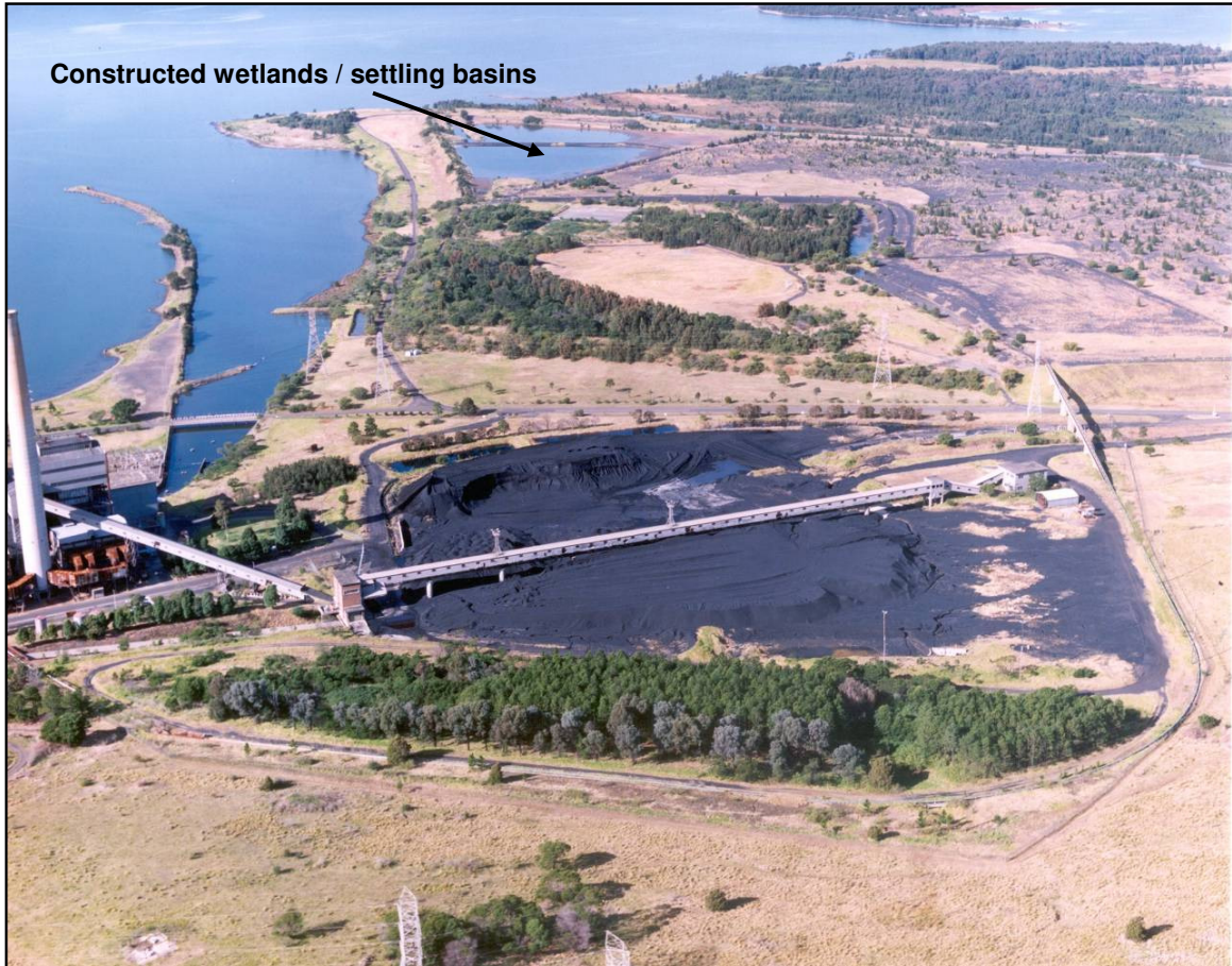
Figure 5: Constructed wetlands when filled with discharged water (Source: TRUenergy)
