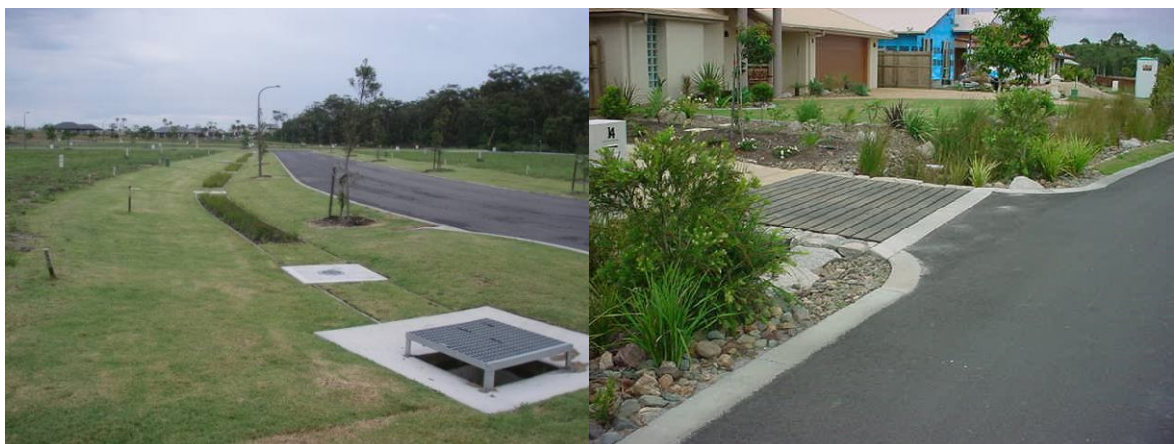
Figure 5-8 Biofiltration Swale Examples
