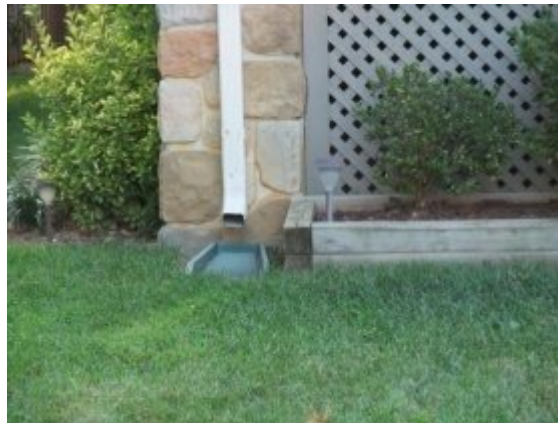
Figure 5-5 Example Disconnection of Roof Surfaces
