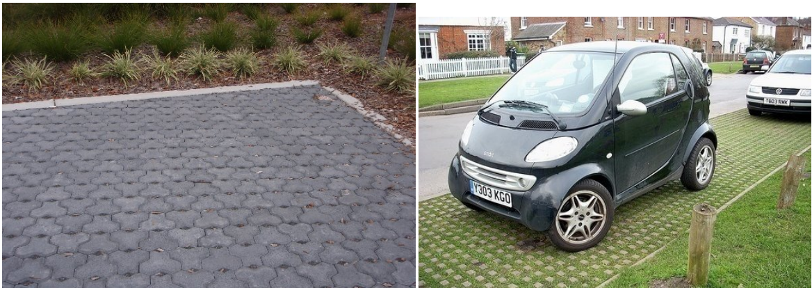
Figure 5-6 Permeable Paving Examples
