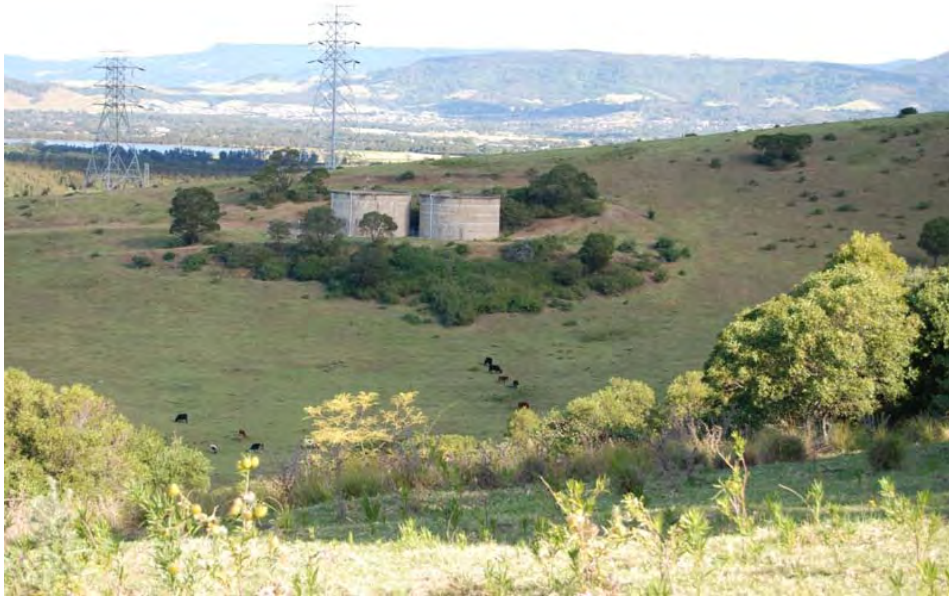
Plate 10: TH8 Concrete Tanks
