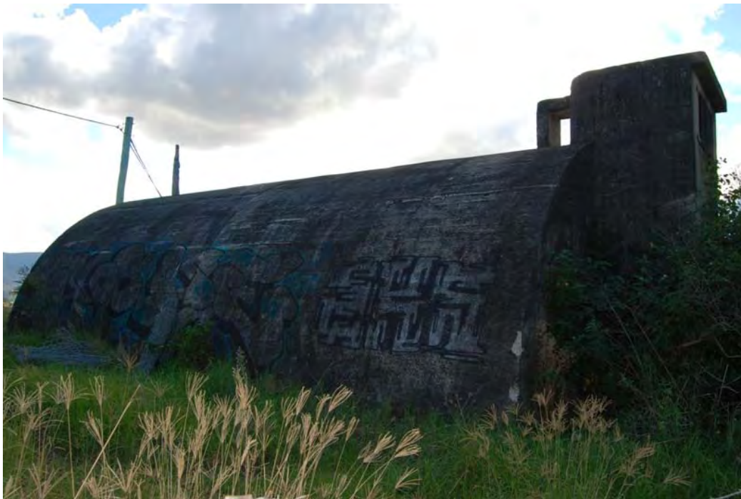
Plate 5: LEP Item 31013 Military Bunker
