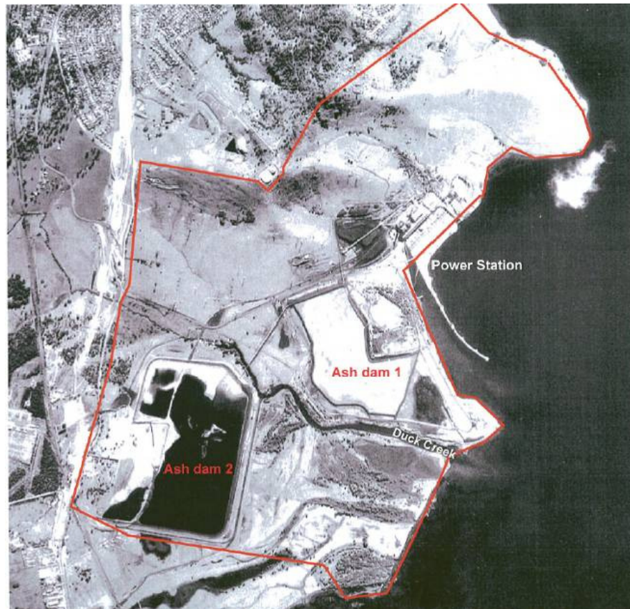
Figure 2.4 Tallawarra Power Station ash dams (1984 photo).
