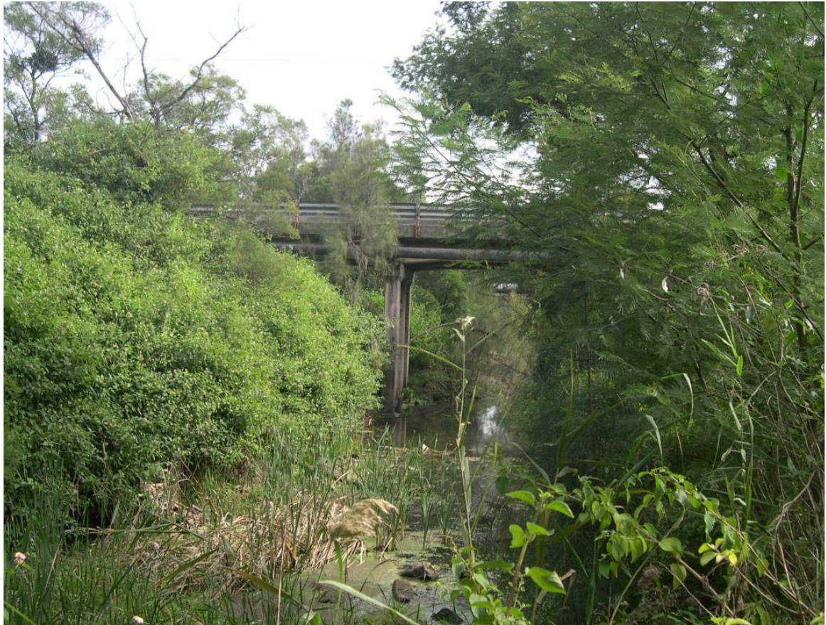
Photo 5: View of Duck Creek at Princes Highway crossing, looking upstream.
