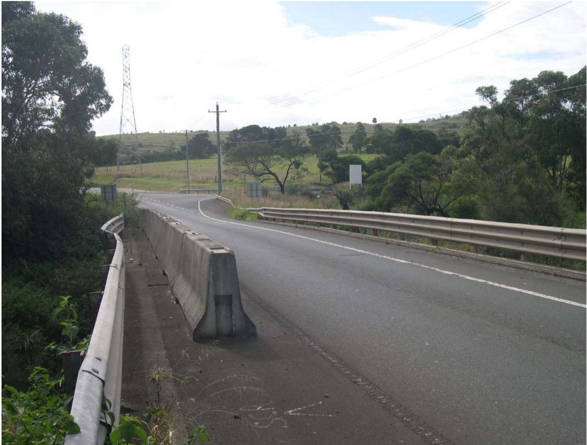
Photo 4: Princes Highway bridge crossing of Duck Creek (Structure No. 11), looking north with Yallah Bay Road intersection in the middle distance.
