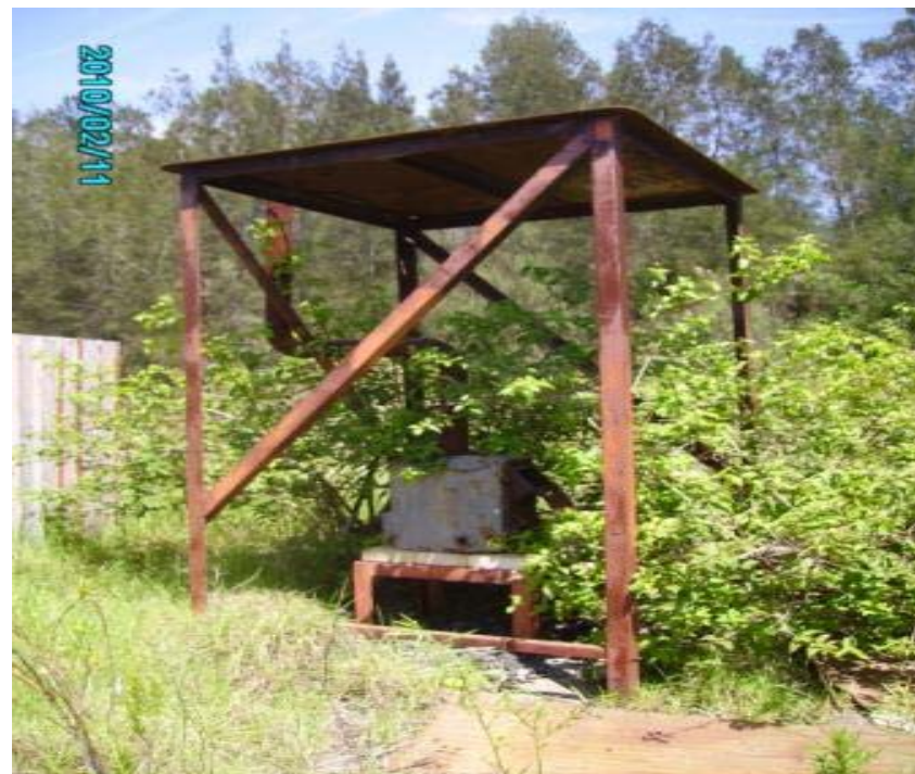
Photo 24 - Looking west at the former coal fired burner in Zone 2(A)
