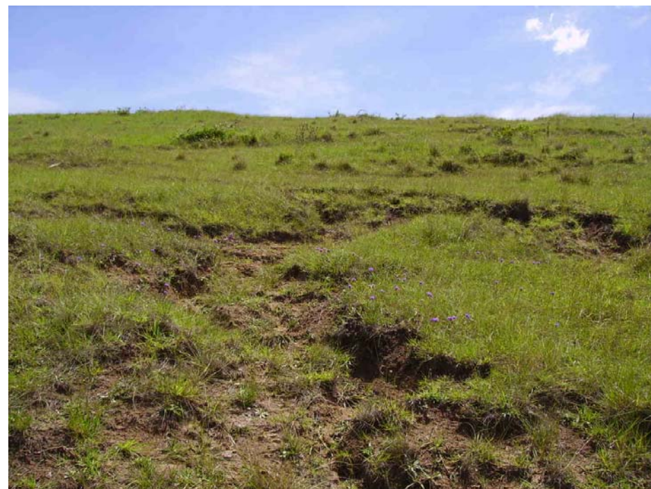
Photo 36E - Erosion and slope instability over steep hillside Zone 2(D).
