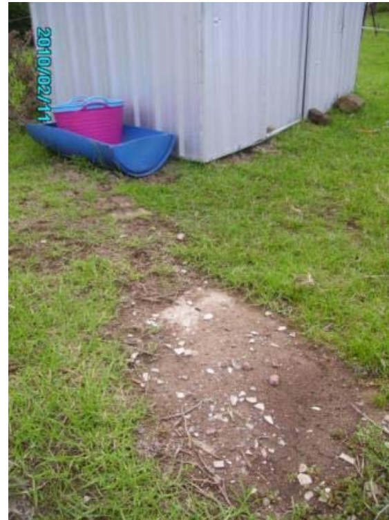
Photo 31 - Disturbed ground surface near the shed indicated in Photo 30. Note the fragments of fibre cement on the ground
