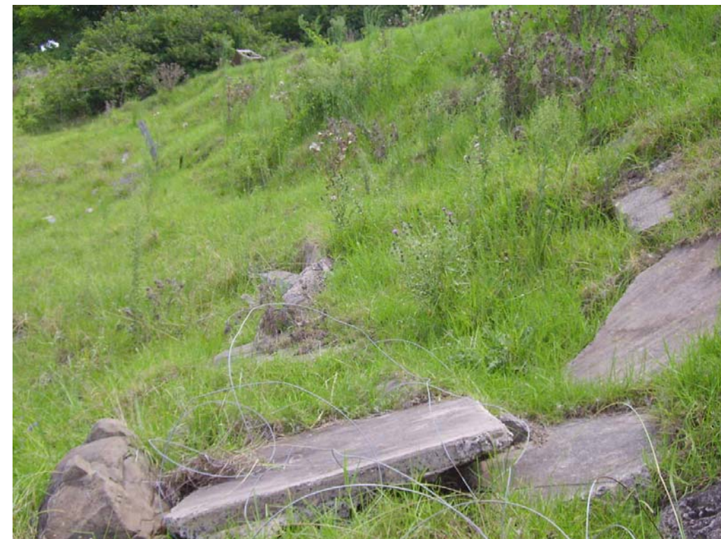
Photo 35B - Piles of concrete and fill mound
