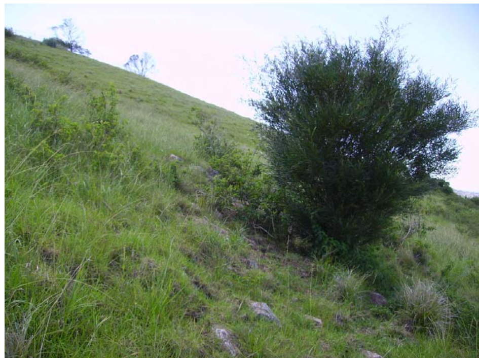
Photo 36D - Loose Latite Cobbles and Boulders on Surface of Steep Slopes at Western End of Zone 2(D). Note irregular surface due to erosion or previous landslide.
