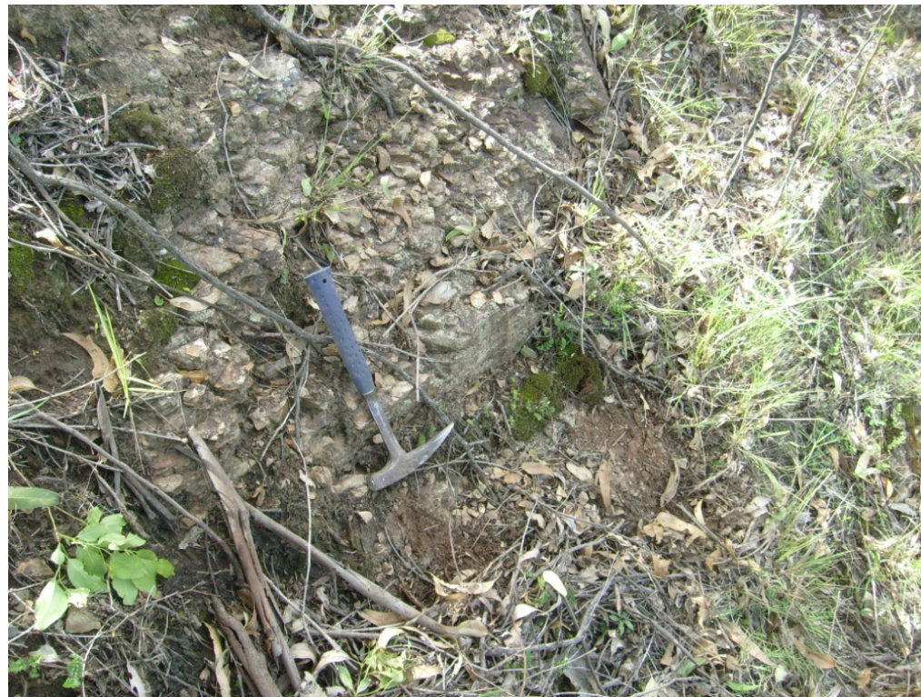
Photo 37C – Outcropping rock observed on the western side of the drainage channel. Noted in Photo 37B, Zone 3(A)
