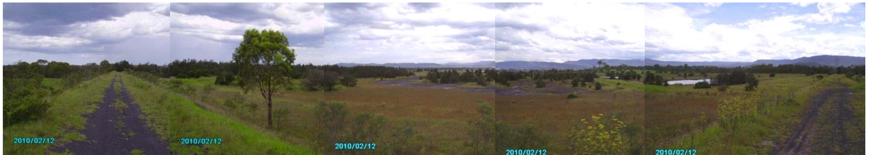
Photo 37A - East to west panoramic view across the northern portion of Zone 3(A) i.e. Ash Pond 3. Note the elevated accessway, with coalwash at the surface
