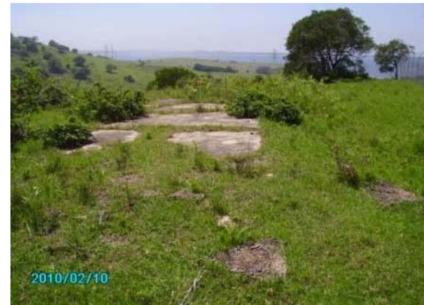
Photo 43 - Concrete slabs in fill soils located on the northern side of the reservoir as indicated in Photo 42
