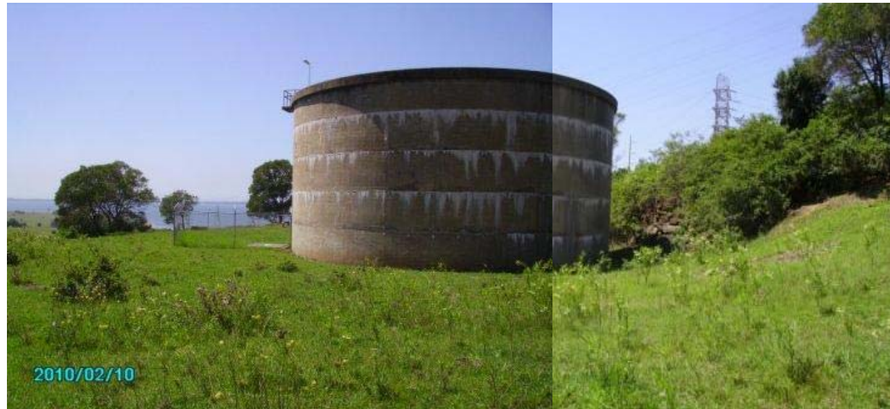
Photo 42 – Concrete Reservoir in the central portion of the Zone. Note the southern side (right-hand side) is cut into the Budgong Sandstone while the northern side lies over of fill
