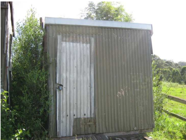
Photograph 35: 20 Corrugated Iron Shed. Locked no access.
