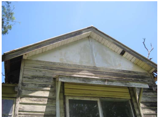
Photograph 24: 11 Garage, External: Red lead paint to roof, cream lead paint to walls.
