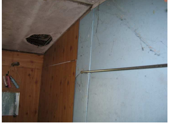
Photograph 6: 01 House, Internal: Cement panels to Bathroom.
