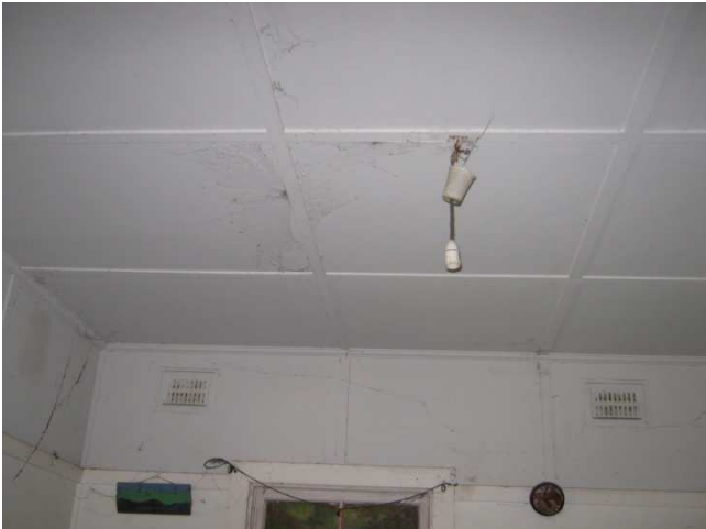
Photograph 17: 01 House, Internal: Cement panel to Sunroom above door.
