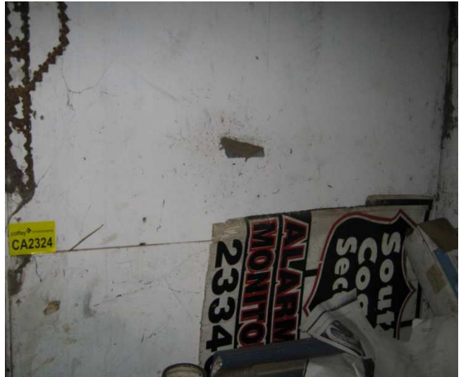
Photograph 38: 13 Tin Shed & Forge, Internal: Cement panels to walls.
