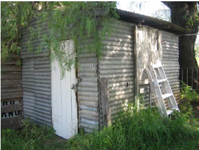
Photograph 29: 14 Tin Shed, External: Cream lead paint to doors & windows.
