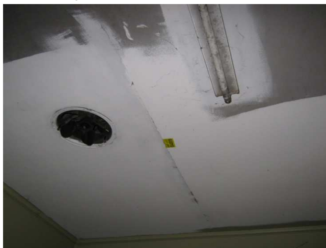
Photograph 12: 01 House, Internal: Cement panels to Kitchen ceiling.
