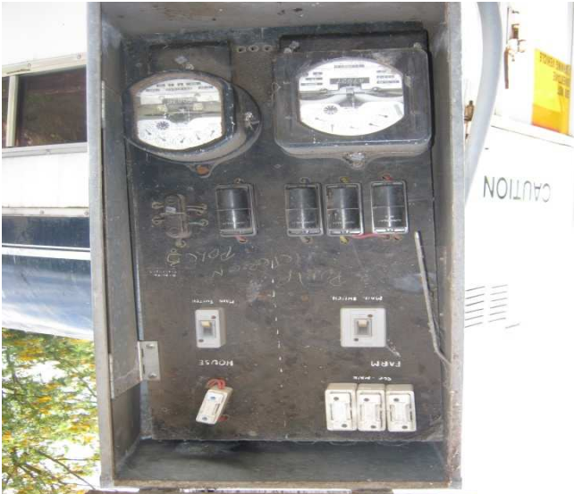
Photograph 27: 12 Stables, External: Zelemite panel to fuse board.
