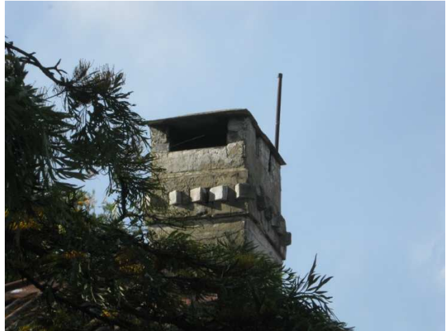
Photograph 52: External Cement panel to house chimney stack.
