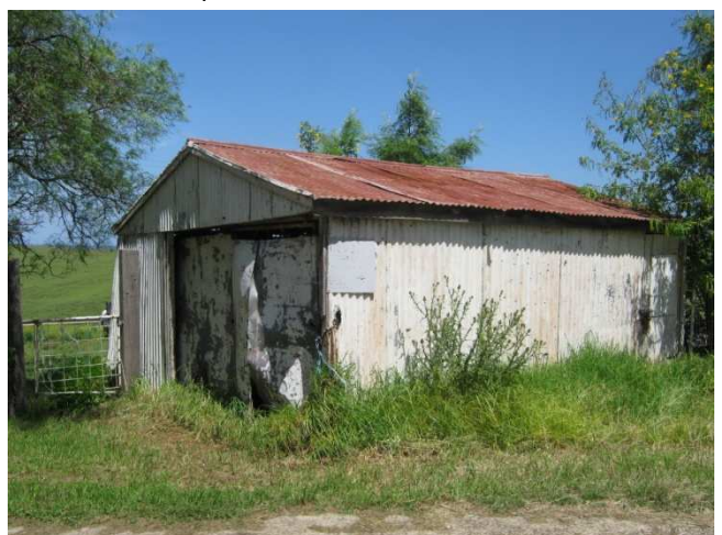
Photograph 24: 11 Garage, External: Red lead paint to roof, cream lead paint to walls.
