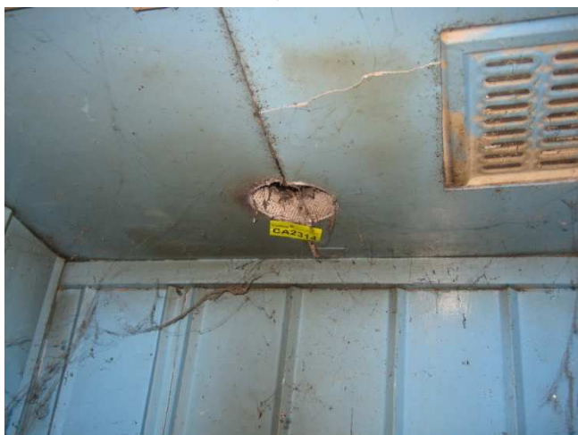
Photograph 11: 01 House, Internal: Cement panels and cloth wrap to Kitchen chimney flue .
