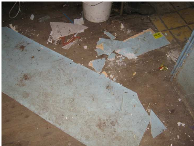
Photograph 9: 01 House, Internal: Cement panel ceiling to Corridor.
