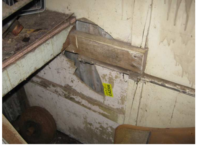
Photograph 2: 01 House, Internal: Car parts store, cement panels.
