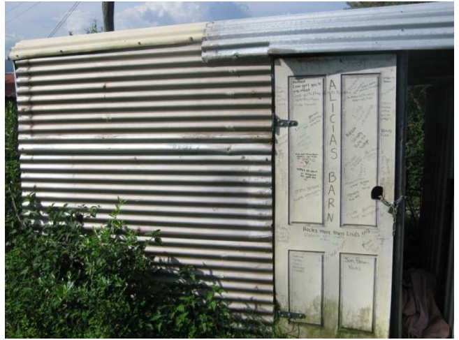
Photograph 38: 23 Corrugated Iron Shed.
