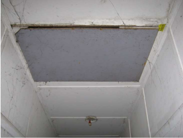
Photograph 15: 01 House, Internal: Cement panels to Bedroom 2 ceiling & walls.
