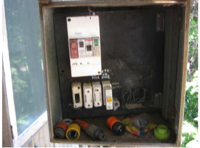
Photograph 18: 01 House, External: Zelemite panel to fuse board.
