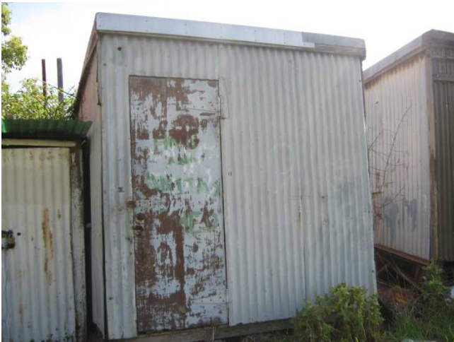
Photograph 33: 18 Corrugated Iron Shed. Locked no access.
