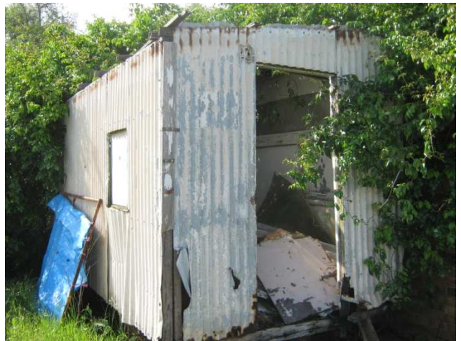
Photograph 42: 27 Corrugated Iron Shed.
