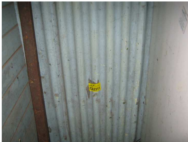
Photograph 10: 01 House, Internal: Cement panels to Kitchen wall.
