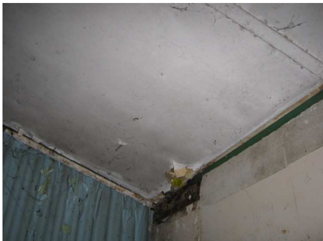
Photograph 11: 01 House, Internal: Cement panels and cloth wrap to Kitchen chimney flue .
