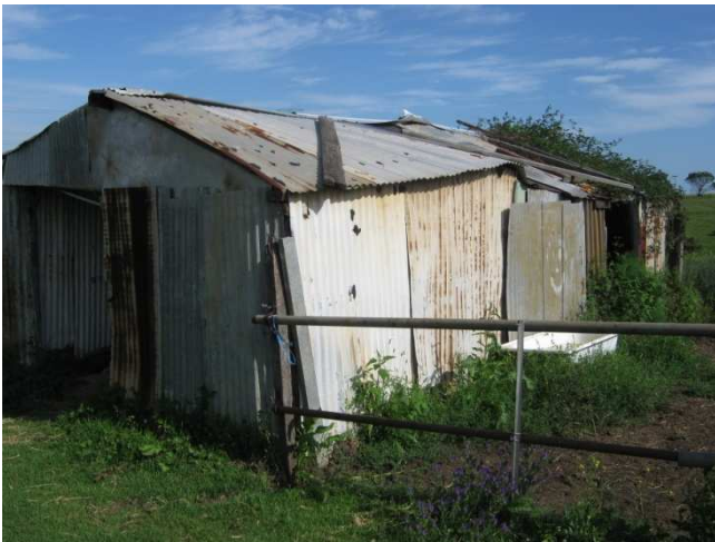
Photograph 41: 26 Corrugated Iron Stables.
