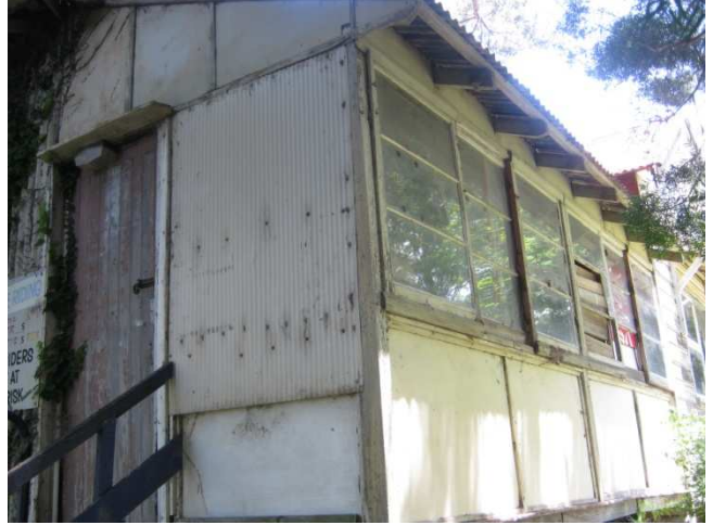
Photograph 22: 01 House, External: Cement panels to gable end.
