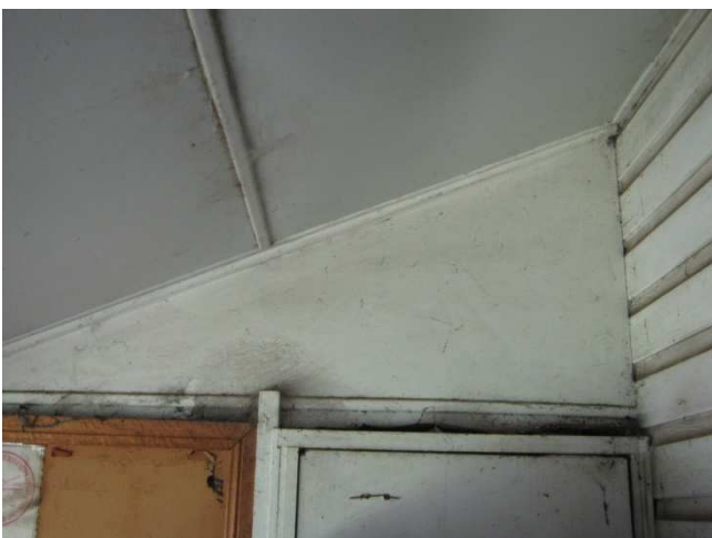
Photograph 17: 01 House, Internal: Cement panel to Sunroom above door.
