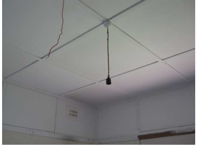
Photograph 16: 01 House, Internal: Cement panels to Office ceiling & walls.
