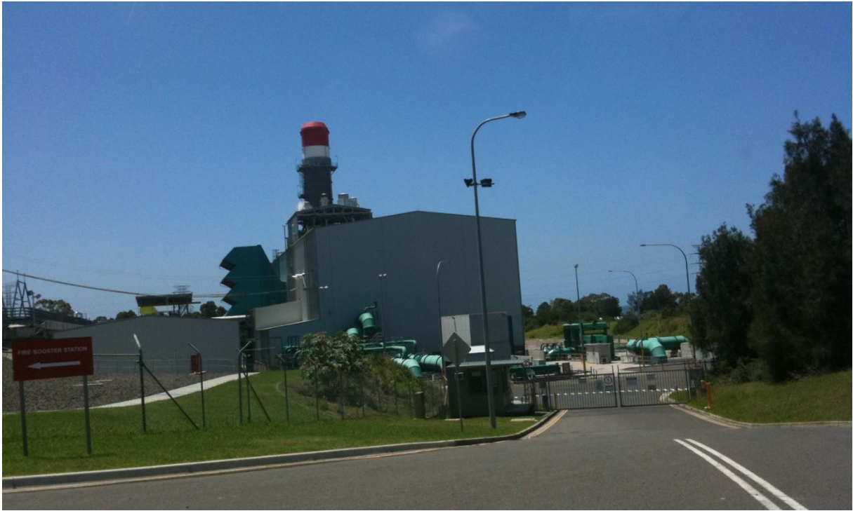
Figure 2. Tallawarra power station
