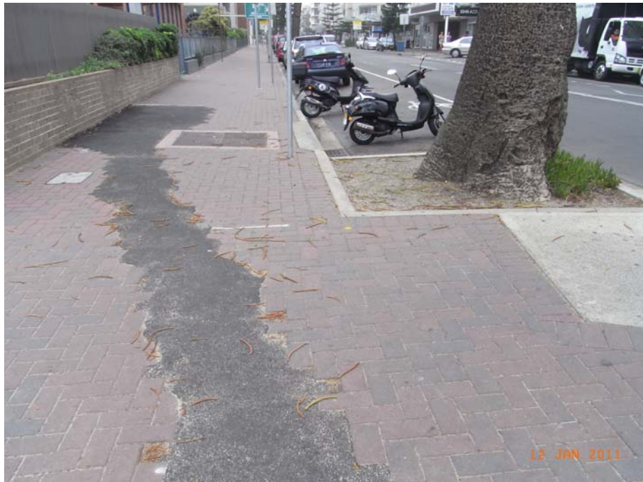
Photograph 2 - Tree # 1 - Illustrating the evidence of recent excavation in close proximity to the tree and within its identified structural root zone.
