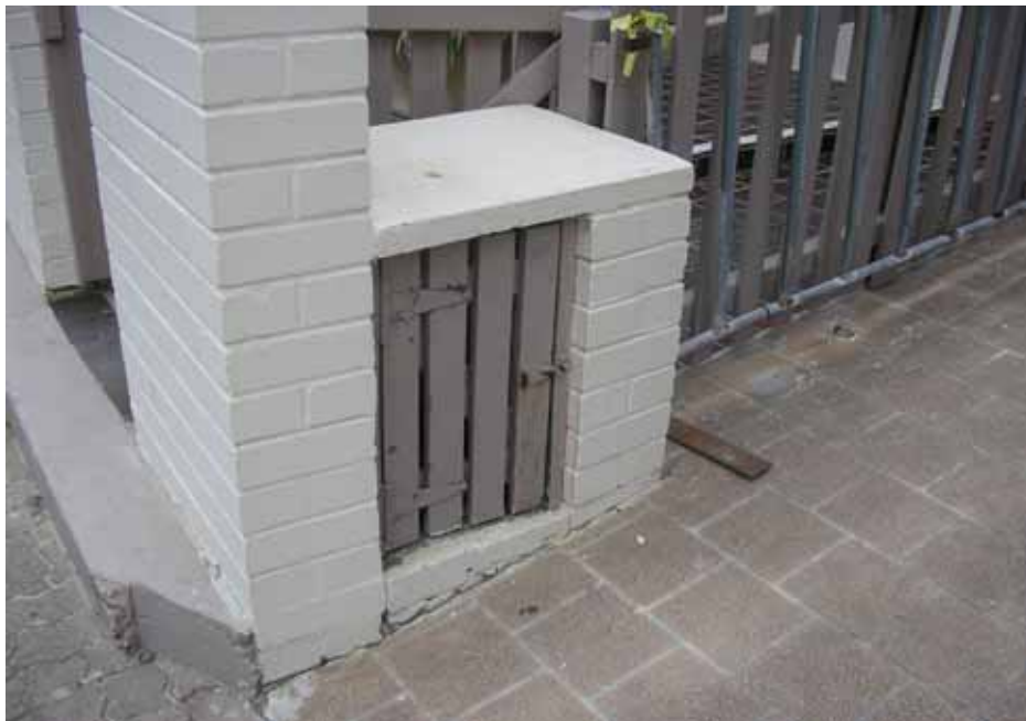
Photograph 29 : Box containing UST fill point in eastern corner of Lot 12, D.P. 1096038, at front of driveway along north east Norman Drummond Bdg 19-21 Wentworth St
