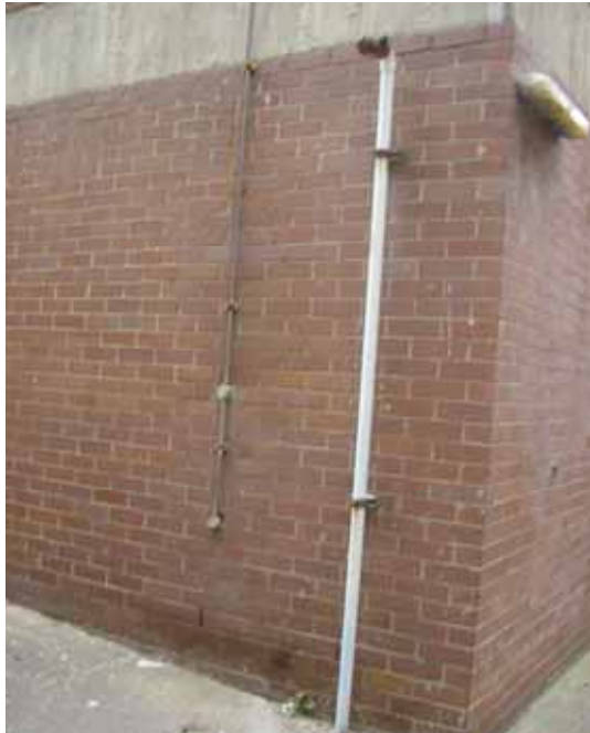
Photograph 33 : Possible breather pipe for UST, on rear (south west) wall of Norman Drummond Bdg 19-21 Wentworth St
