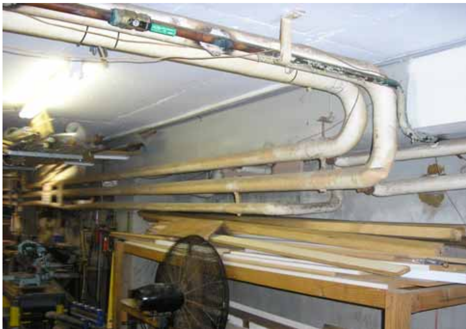
Photograph 9 : Workshop beneath Elsie Hill Bdg, pipes with asbestos lagging
