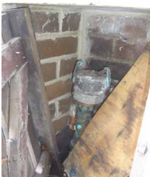
Photograph 30 : UST fill point in above box
