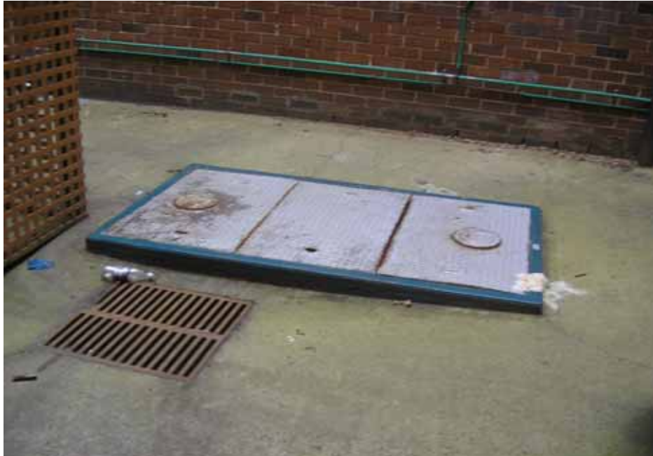
Photograph 38 : Grease trap in rear (south west) courtyard of Norman Drummond Bdg 19-21 Wentworth St
