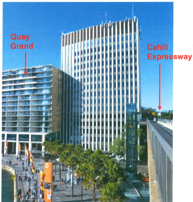
Figure 3: The existing building situated between the Quay Grand and the Cahill Expressway (Source: Proponent's EA)
