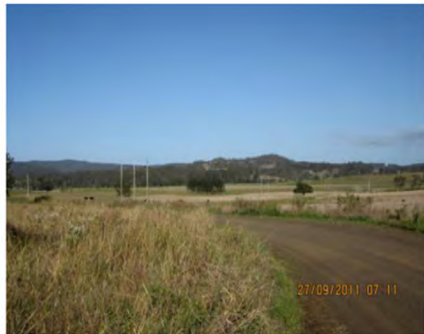
Existing angle (AP60) and transmission line looking south-west from Ellems Bridge Rd
