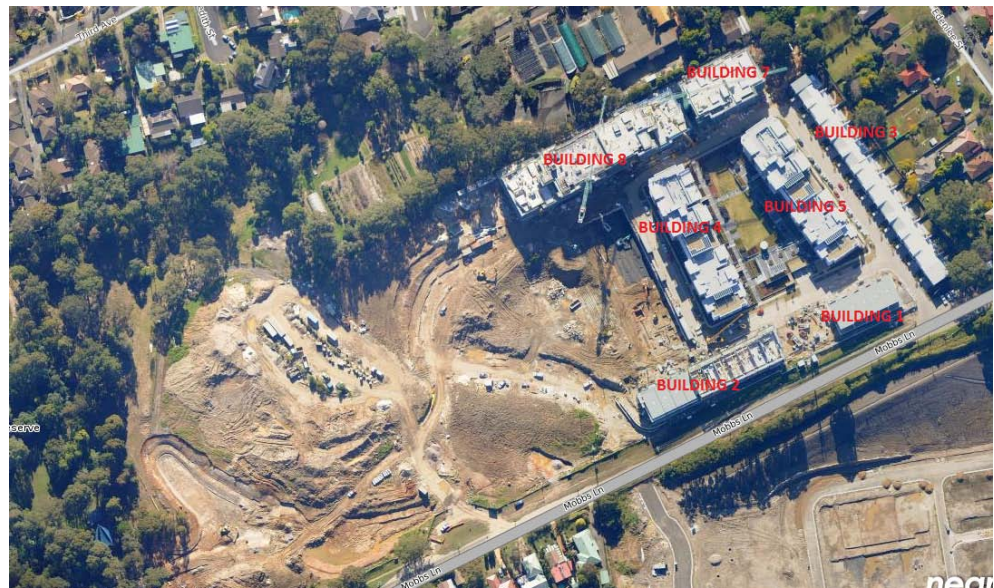
Figure 6: Subject site, currently under construction
