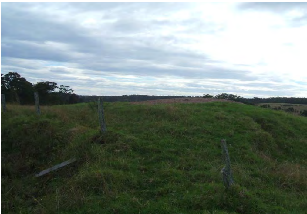
Photo plate 20 - Dam wall to the north east of Homestead
