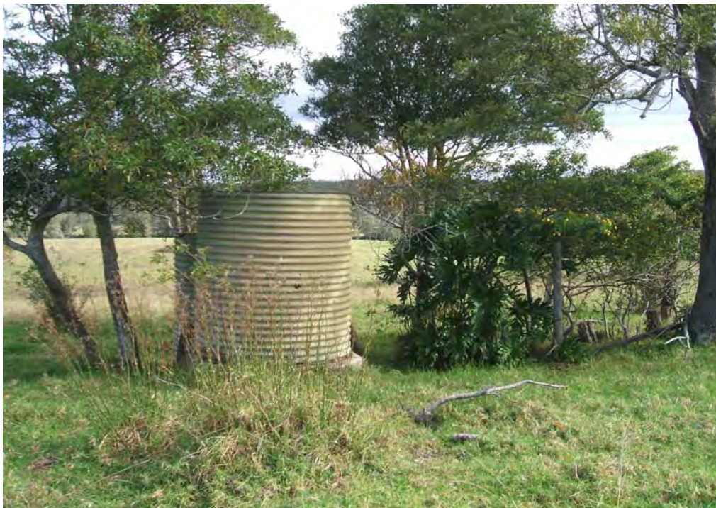
Photo plate 15 - Tanks adjacent to Former Homestead
