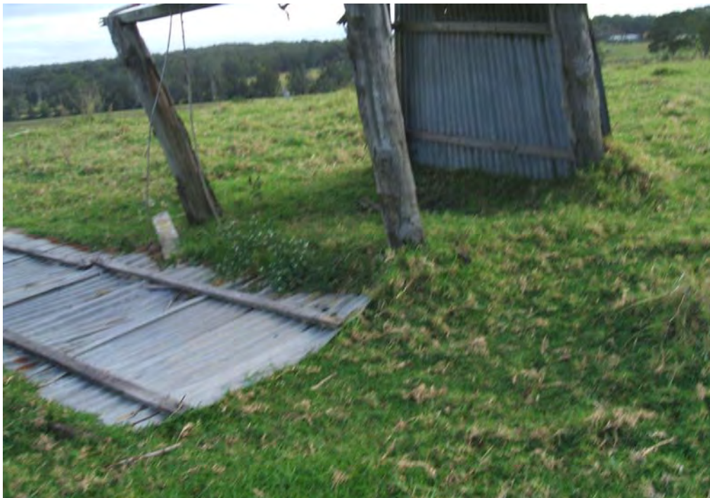
Photo plate 26 - Smaller structure near collapsed structure
