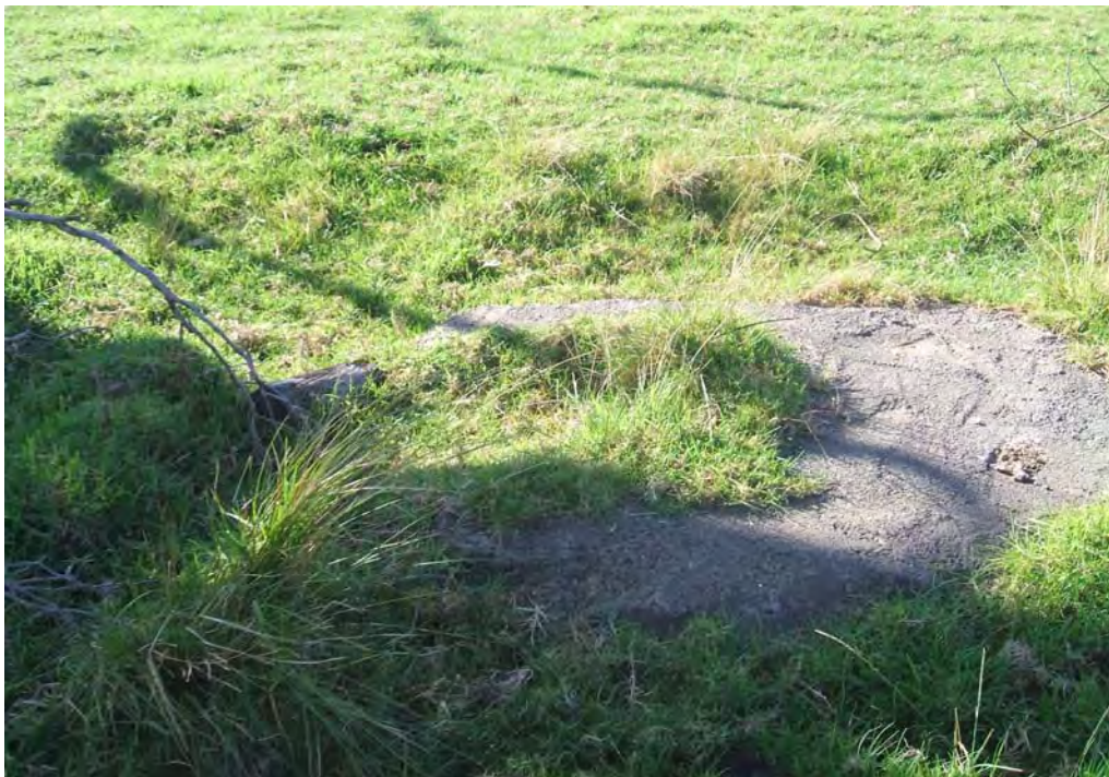
Photo plate 8 - U Shaped concrete slab
