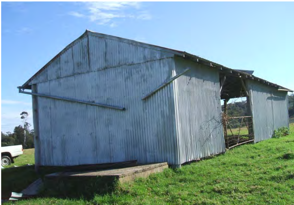
Photo plate 7 - Concrete pit behind Dairy shed
