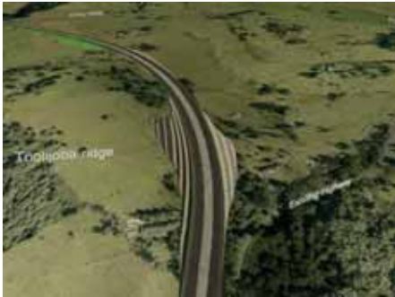
Figure 6.3 Significant cutting at Toolijoo Ridge
