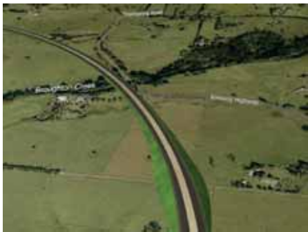
Figure 6.9 Large embankments crossing the Broughton Creek floodplain
