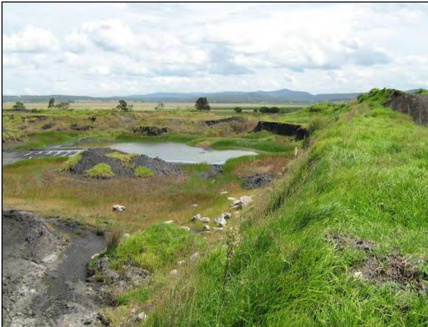
Figure 3: Looking west along the northern wall of the excavation. Leached salts are evident in sporadic locations at the base of the excavation
