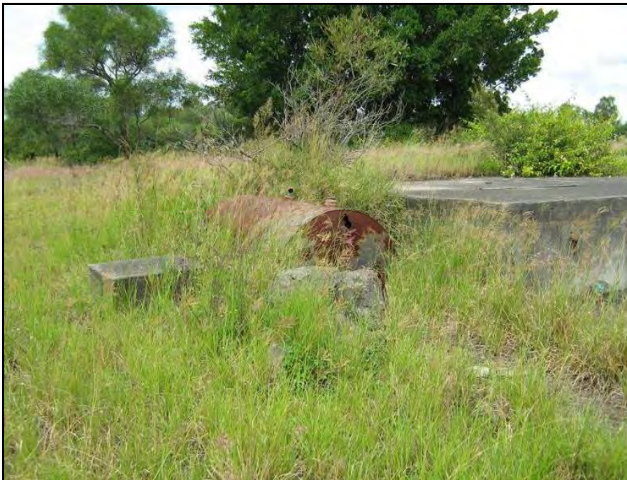
Figure 4: Abandoned former Underground Storage Tank located adjacent to a concrete platform in the south-eastern portion of the site
