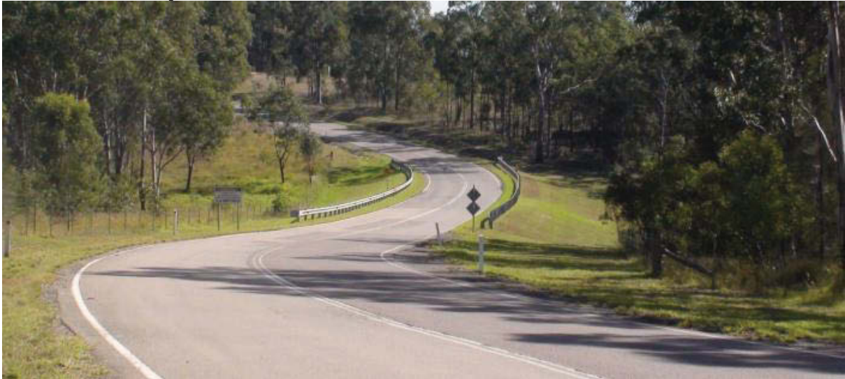
Plate 6 Drayton Mine Access Road
