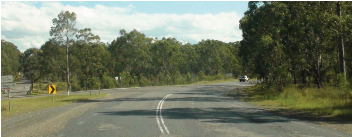
Plate 9 Thomas Mitchell Drive near intersection
