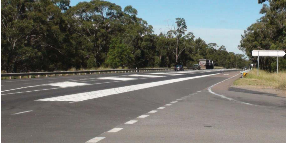
Plate 7 New England Highway near intersection
