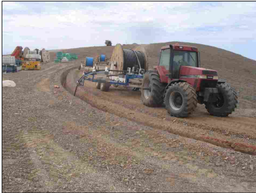
Image 3.7 Laying underground electrical cable within the road network
