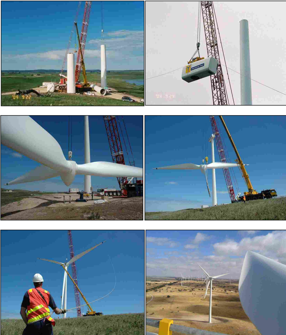
Image 3.11 A range of typical turbine erection photographs
