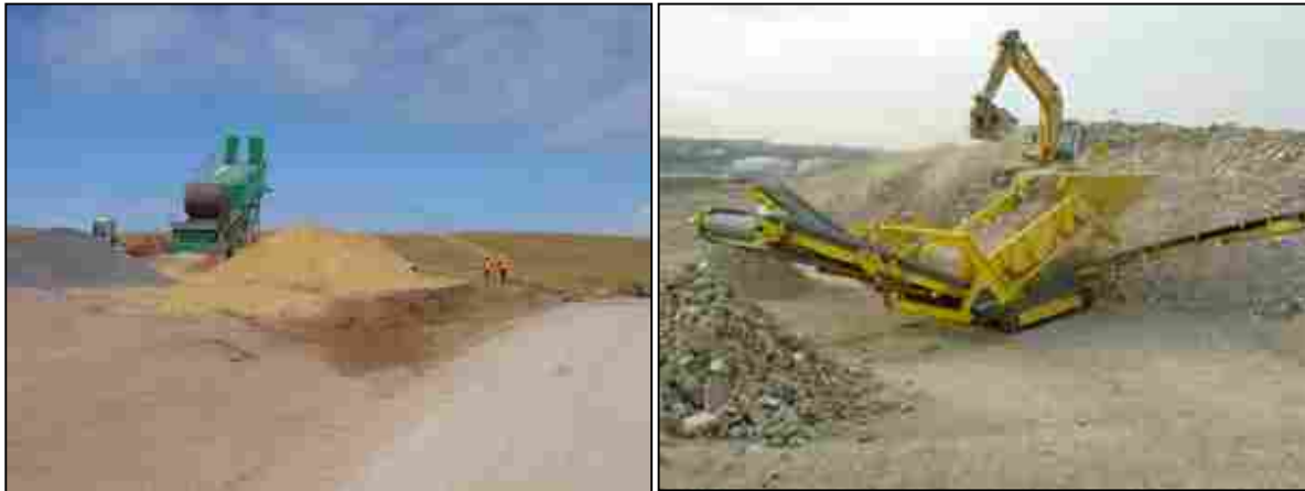
Image 3.9 Temporary on-site concrete batching plant and rock crusher
