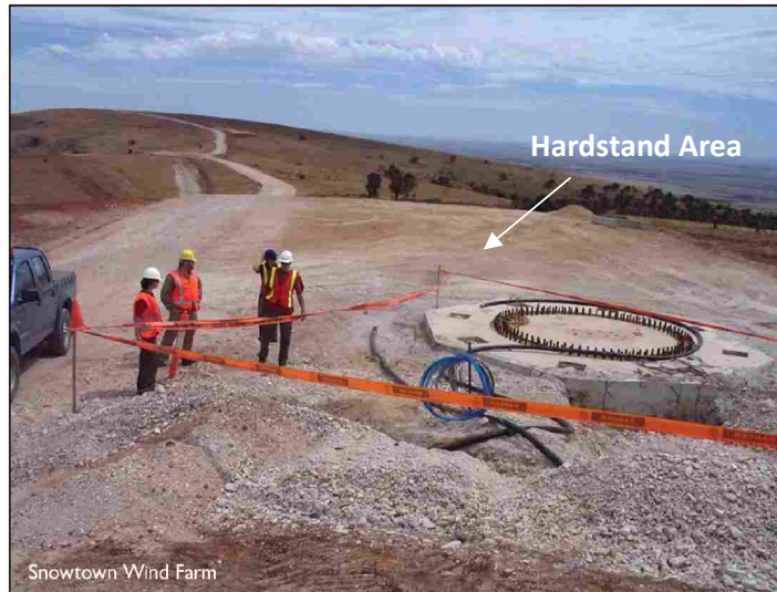
Image 3.3 Typical hardstand area adjacent to a rock anchor footing
