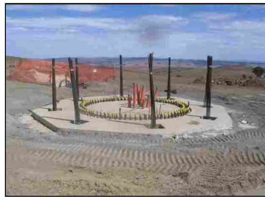
Image 3.2 Typical gravity (left) and rock anchor (right) footings
