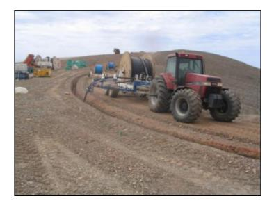
Image 7: Laying underground electrical cable within the road network Photo Courtesy: Wind Prospect CWP
