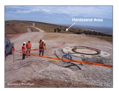
Image 3: Typical hardstand area adjacent to a rock anchor footing Photo courtesy: Wind Prospect CWP
