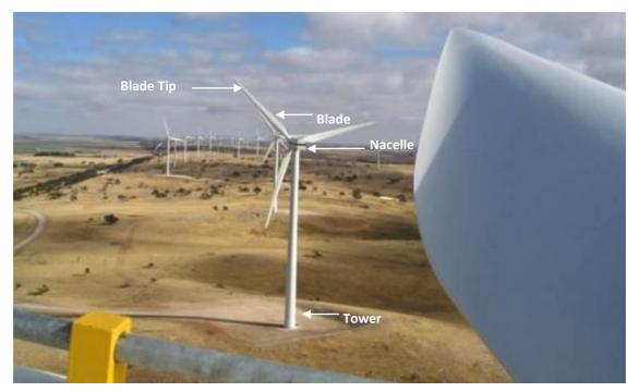
Image 1: Component Parts of a wind turbine Photo courtesy: Wind Prospect CWP
