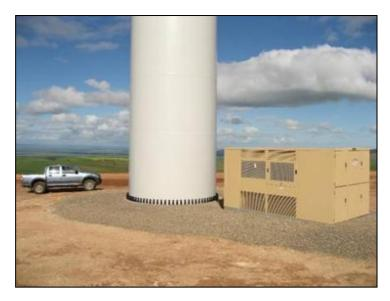
Image 5: Transformer adjacent to wind turbine Photo Courtesy: Wind Prospect CWP
