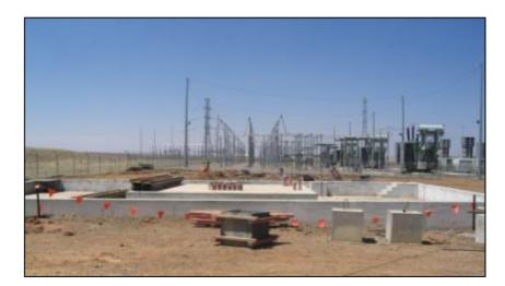
Image 10: Transformer foundation (foreground) and electrical substation and switchgear infrastructure (background). Photo Courtesy: Wind Prospect CWP
