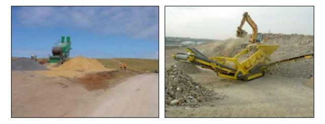
Image 9: Temporary on-site concrete batching plant and rock crusher Photo Courtesy: Wind Prospect CWP
