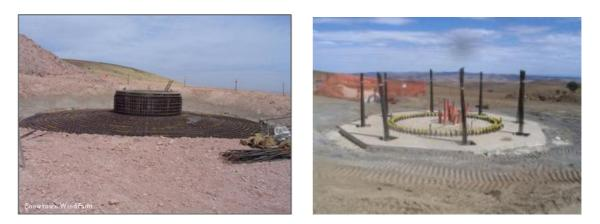
Image 2: Typical gravity (left) and rock anchor (right) footings Photo courtesy: Wind Prospect CWP
