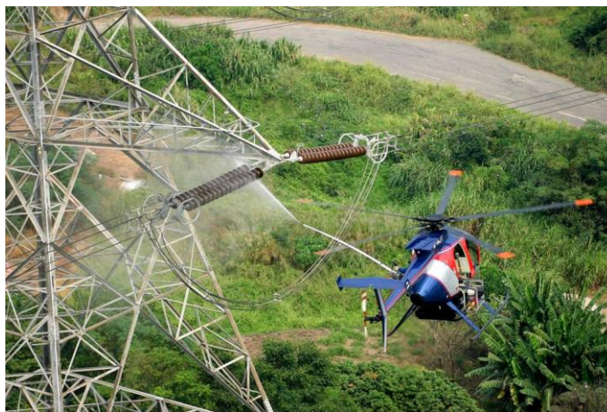
Washing insulators using a MD 500 helicopter.
