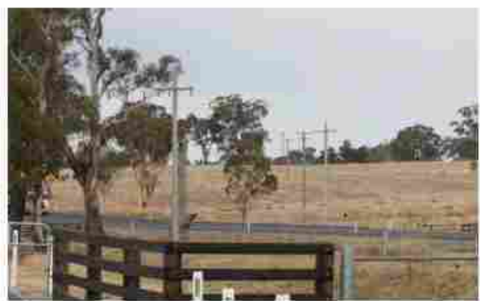
Existing Powerlines- Castlereagh Highway
