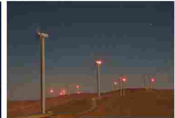
Example of obstacle lighting at Waubra Wind Farm (Source: Flickr)
