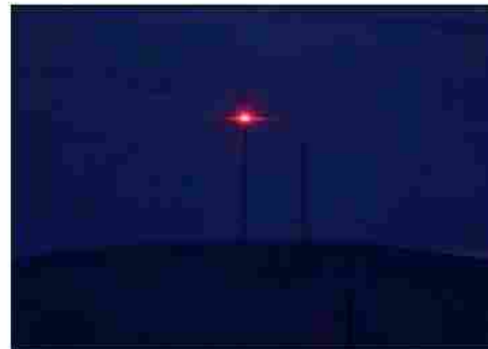
Example of obstacle lighting at Waubra Wind Farm (Source: Flickr)
