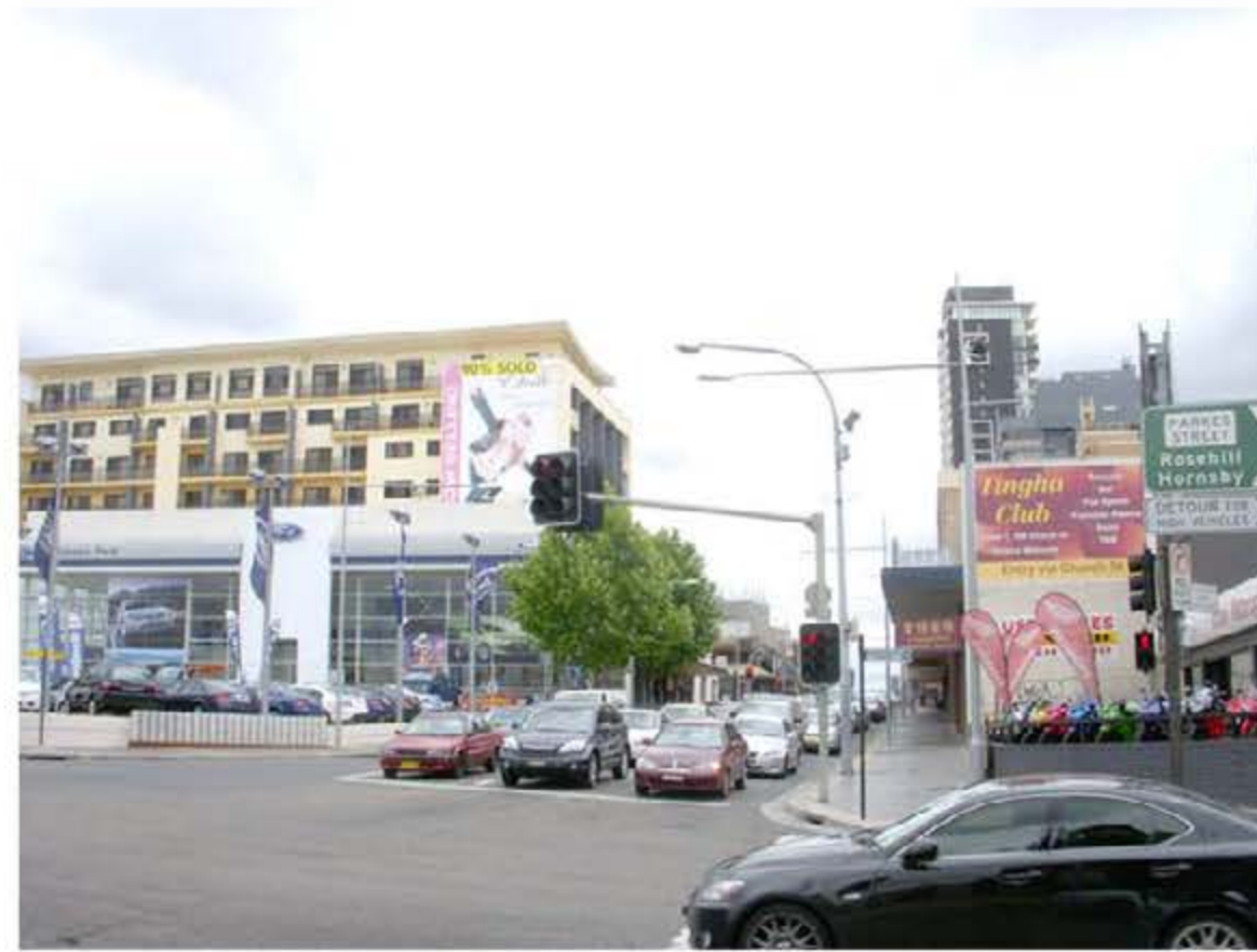
Existing View From Church St looking North
