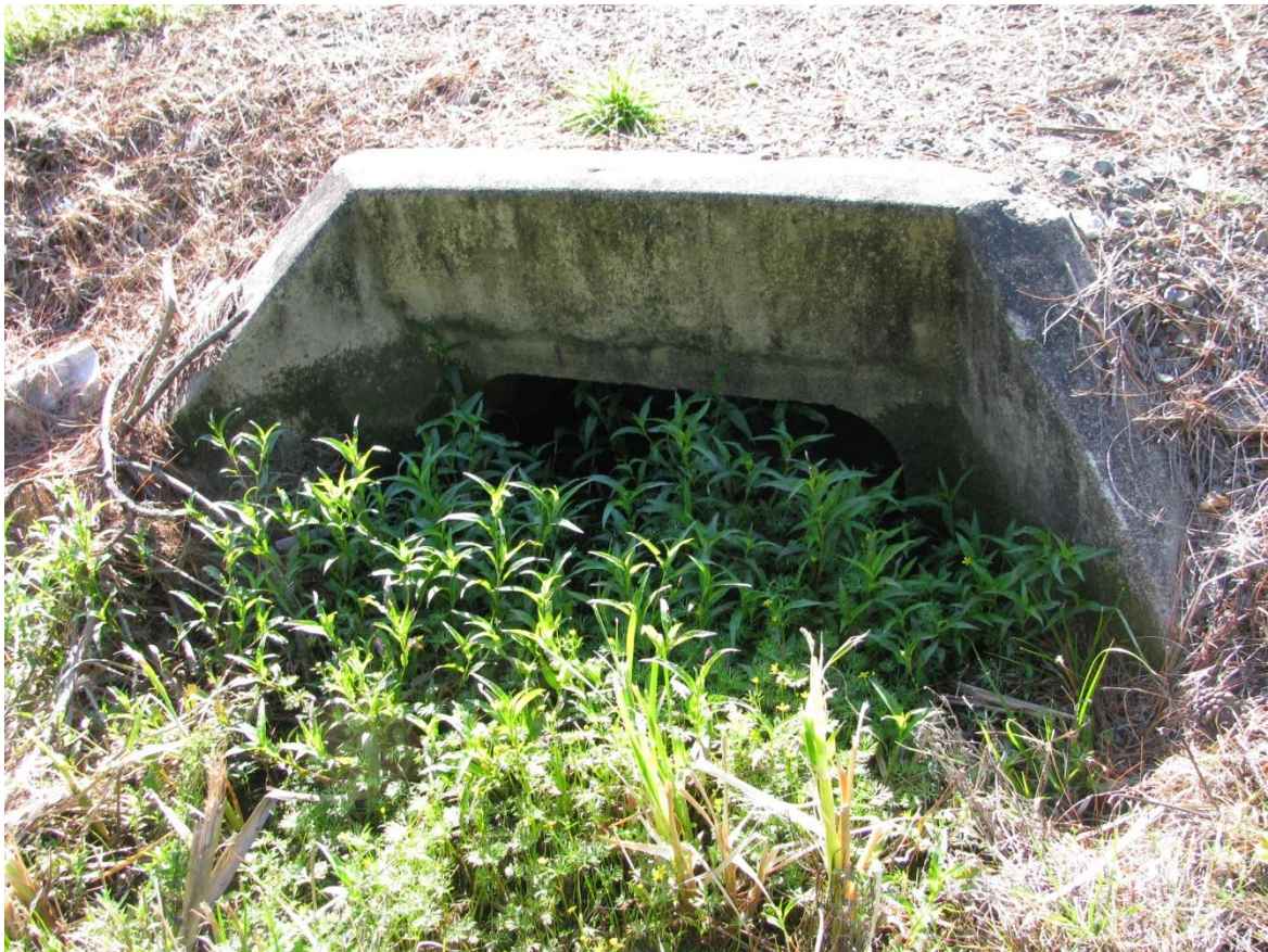
Photograph 2 – Small existing culvert will be removed adjacent to Riverside development
