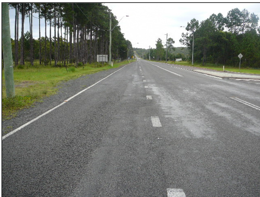
Photo 1 View west along Myall Street showing typical cross section
