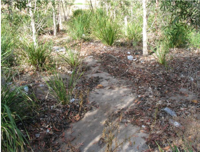
Figure 1 Litter collecting on the surface of a biofilter
