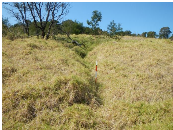
Plate 5: View east of erosion gully associated with a contour bank
