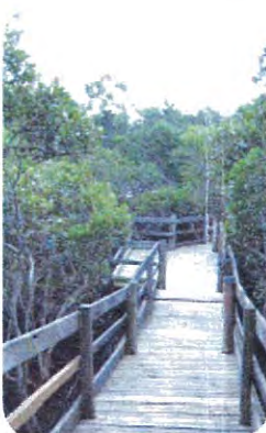
Upgrade existing boardwalk > Woollooware Bay Mangrove Boardwalk
