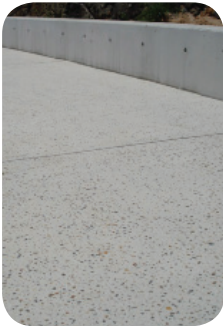
In situ concrete footpath with exposed aggregate > ASPECT image library
