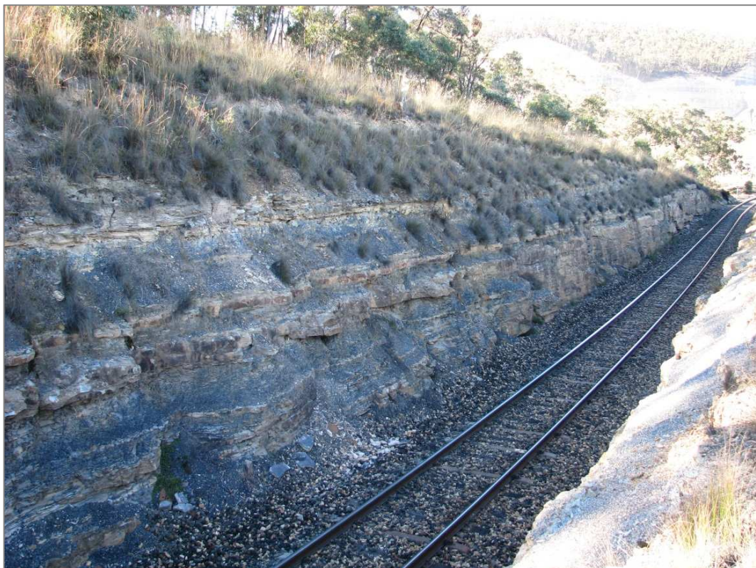
Figure 2a – Photograph of the railway cutting undamaged by blasting at 30m
