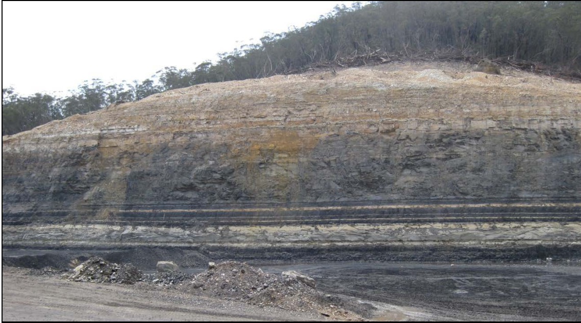
Figure 2 Cullen Valley showing a stable, 80 m highwall face cut at an angle of approximately 80°.
