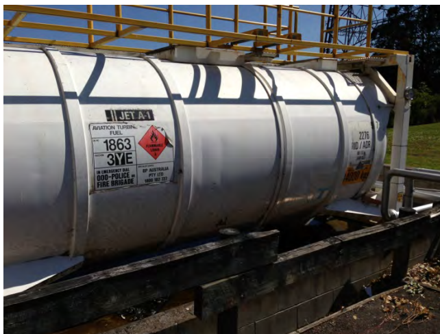
Photo 4 –AST located to the east of the helipad.
