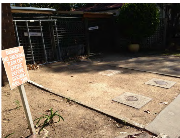
Photo 1 – Dip points and Danger sign associated with USTs tanks 2 and 3.
