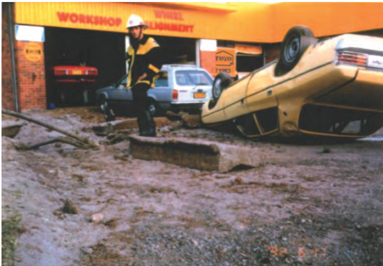
Welding the tank vent pipe caused vapours in the tank to explode.
