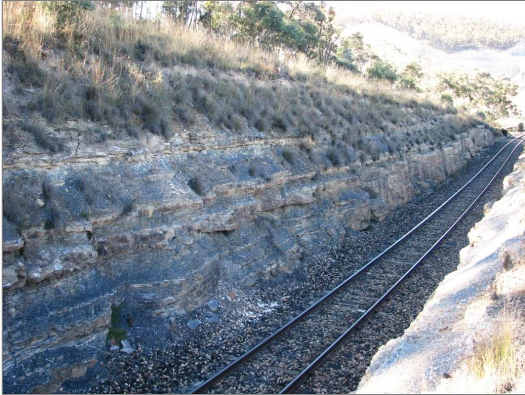
Figure 3a – Photograph of the railway cutting undamaged by blasting at 30m
