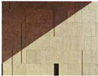
EXTERIOR WALLS - SANDSTONE
