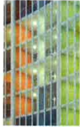
LOUVRED VENTILATION TO CORRIDORS
