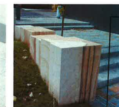
EXPOSED AGGREGATE CONCRETE PAVING
