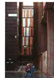
WALL TREATMENTS - TIMBER COMPOSITE PANELS + ALUMINIUM CLADDING
