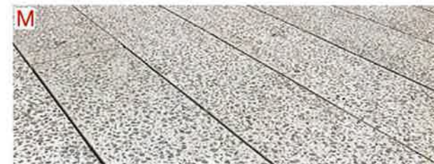
Large format concrete paving
