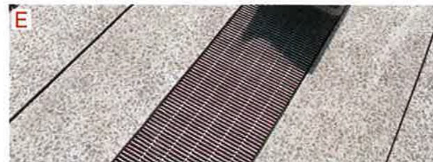
Steel Tree Grill flush with Paving
