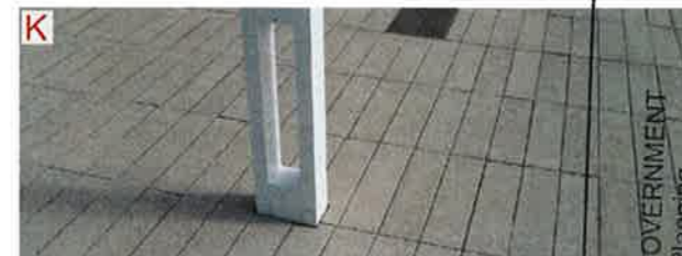
Small format concrete paving
