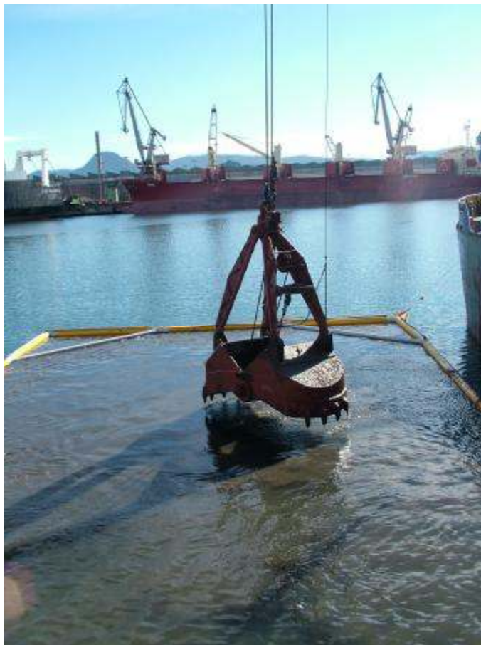
Photo 3.2 Close up view of grab dredger operating within a turbidity curtain
