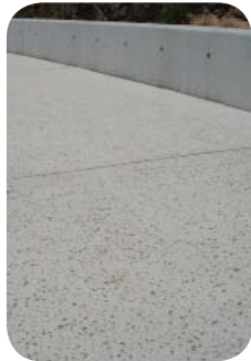
In situ concrete footpath with exposed aggregate > ASPECT image library
