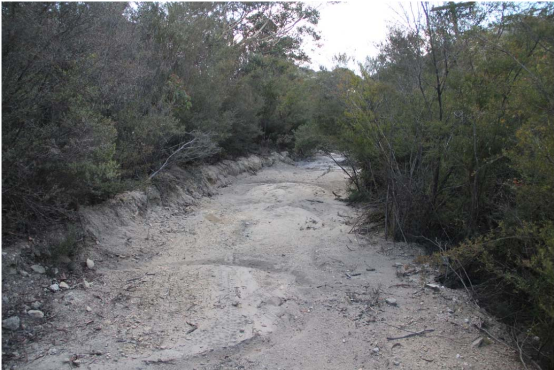
Plate 7 Runoff from track use Adjacent to Plate 2 site
