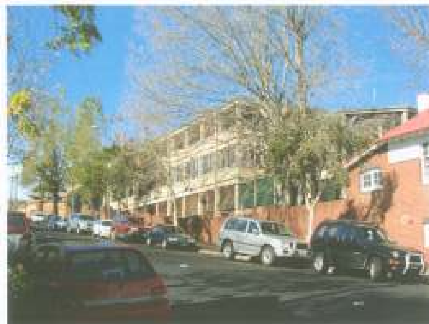
Figure 10 Red brick wall along Burton Street.
