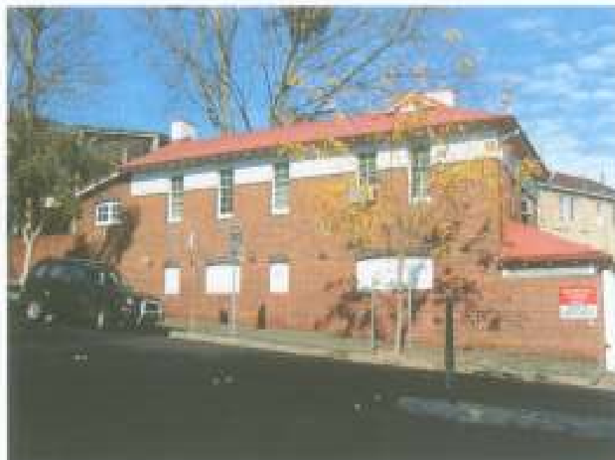
Figure 8 Former Kitchen building from Burton Street
