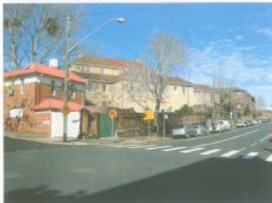
Figure 12 Rear additions viewed from Bourke Street. Note the highest visible roof point is of the third floor addition to the original Cartas House (B, 62 msl).
