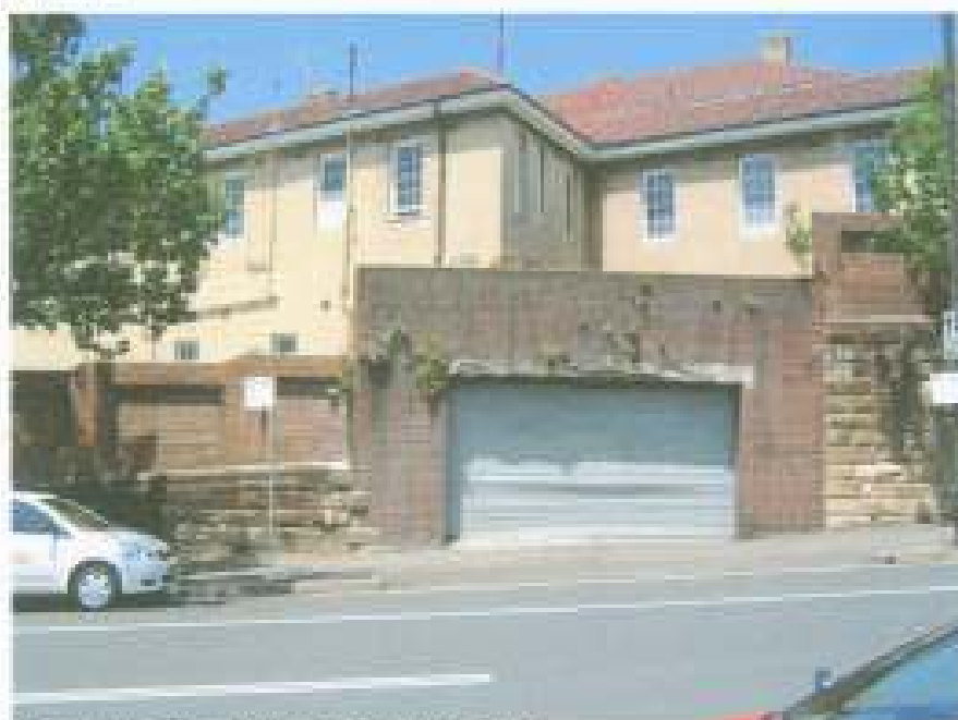
Figure 11 Mix of wall styles along Bourke Street
