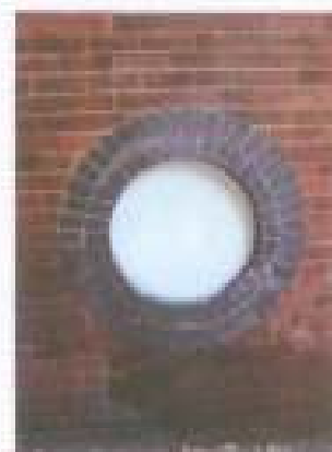
Figure 58: Former window along the Burton Street (north) side (Source: Graham Brooks & Associates, July 2006)
