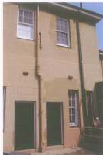
Figure 38: Rear of the addition, showing two doors at the west end, with basement area being the lower level. (Source: Graham Brooks & Associates, July 2008)
