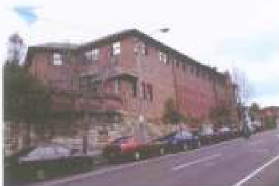
Figure 1: The point where the Carfax wall meets the walls of the former Darlington Police Station. (Source: Graham Brooks & Associates, July 2006)
