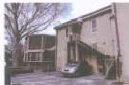
Figure 31 The later 1930s extensions, looking north inside the property boundary. The roof is a rendered concrete faux stone with corrugated steel roof (Source: Graham Brooks & Associates, July 2008)
