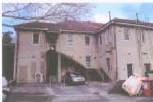
Figure 39 View (Source: Graham Brooks & Associates, July 2008)
