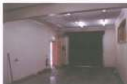
Figure 65 Interior lower level garage space. Nothing appears to connect from former area (Source: Graham Brooks & Associates, July 2006)
