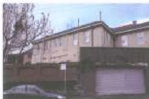
Figure 19: View of the west facade of the property where the 1888 intervention in the wall was checked for the garage and showing the c. 1930 building additions for skillets, stone etc. (Source: Graham Brooks & Associates, July 2008)
