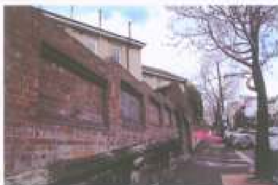
Figure 12: The original stone retaining walls, capped to brick, having probably existed in the 1820s. It seems to have already been in place when the interventions were made for the garage and driveways along this side. (Source: Graham Brooks & Associates, July 2008)
