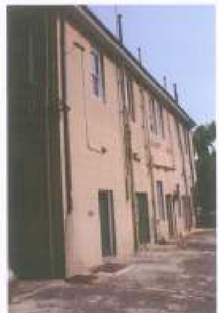
Figure 41 The later 1900s additions at the west side (rear) of the property (Source: Graham Brooks & Associates, July 2008)
