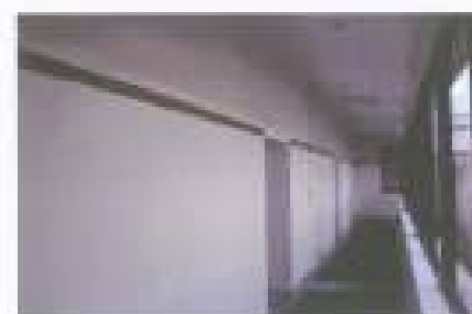
Figure 32 Inside the rear extensions adjacent to the southwest toilet facility which comprises a large part of the corner of the building. The interior finish is very simple and appears to have had a number of columns supporting (Source: Graham Brooks & Associates, July 2008)
