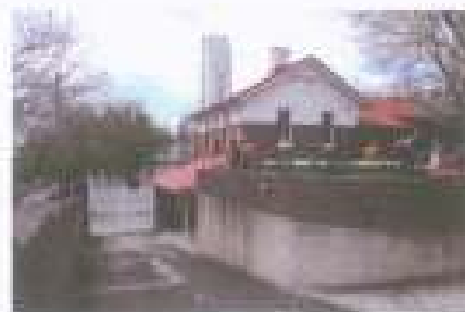
Figure 55: View down the ramp to Burton Street (Source: Graham Brooks & Associates, July 2006)
