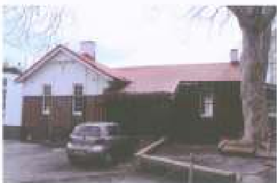
Figure 54: The level of the ground at the top of the ramp and at the first floor level of the old kitchen facility, which served as a flat for individual tenement for some time. (Source: Graham Brooks & Associates, July 2006)
