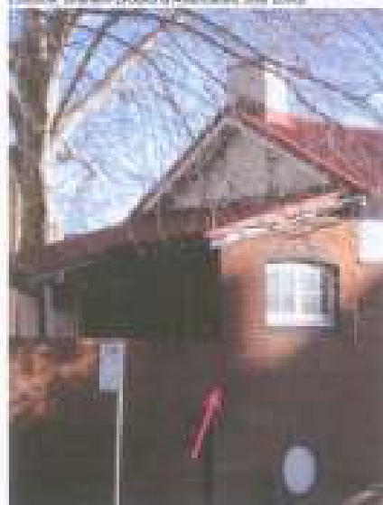
Figure 100. Detail view of the north side of the old kitchen facility taken from Burton Street and showing intersection with brick wall (Source: Graham Brooks & Associates, July 2008)
