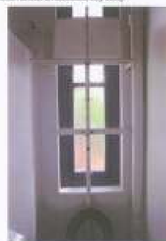
Figure 47 Interior of the washroom facilities (Source: Graham Brooks & Associates, July 2008)
