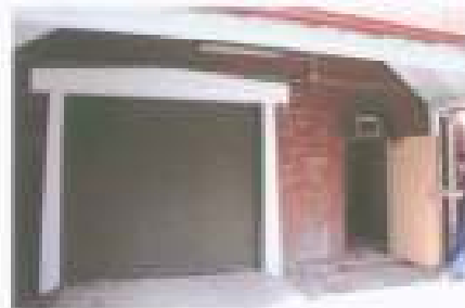
Figure 63 Lower level of the old kitchen facility showing the connection to garage (Source: Graham Brooks & Associates, July 2006)
