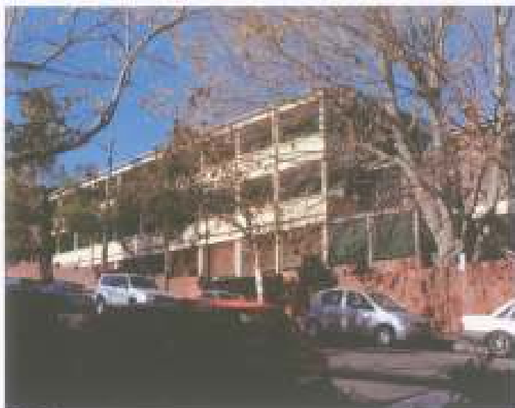
Figure 26: View of the 1980s building, and showing a perimeter fencing/wall arrangement which seems consistent with that era. It is not clear what complicates the foundation for this wall. (Source: Graham Brooks & Associates, July 2008)
