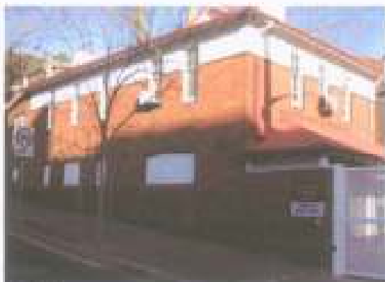
Figure 52: View of the southwest corner, old kitchen facility, adjacent to security entrance gate (Source: Graham Brooks & Associates, July 2006)
