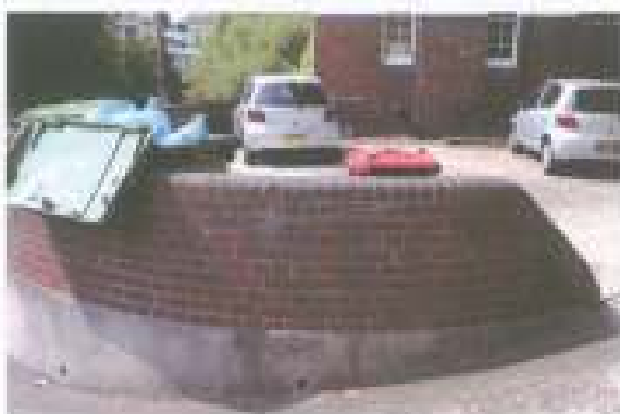
Figure 62 The curved retaining wall counting wheel up from Butler Street (Source: Graham Brooks & Associates, July 2006)
