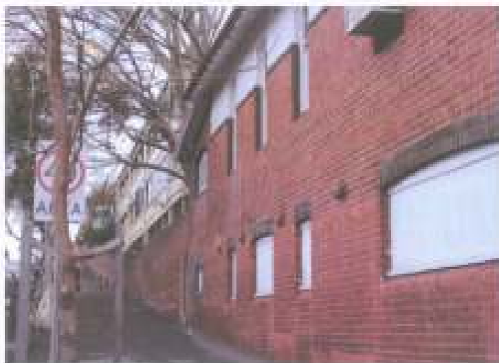
Figure 28: View looking west up Burton Street from the corner of the old kitchen facility. (Source: Graham Brooks & Associates, July 2008)
