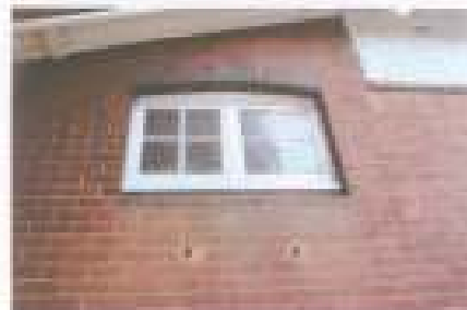
Figure 57: Window along the Burton Street (north) side (Source: Graham Brooks & Associates, July 2006)
