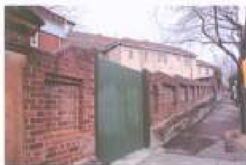
Figure 12: View looking south up Bourke Street showing brick wall and stone foundation retaining wall. The brick wall is probably 1820s and was already in place when the 1870 plans were drawn up. (Source: Graham Brooks & Associates, July 2008)
