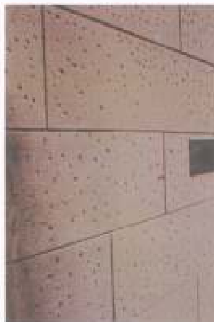
Figure 39: Detail of the face stone work/courtyard wall. (Source: Graham Brooks & Associates, July 2008)
