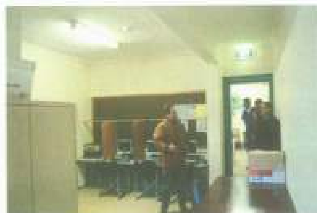
Figure 73 The interior of the Carfax Cottage has undergone extensive modification and re-configuration and introduction of various services. This supports both work and removal. (Source: Graham Brooks & Associates, July 2008)
