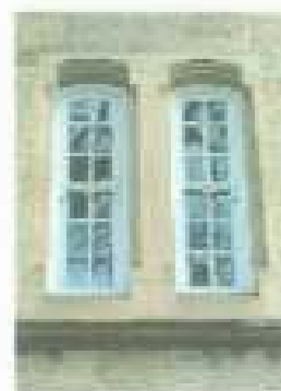
Figure 84 Original Regency style window openings and sculptured stonework (Source: Graham Brooks & Associates, July 2016)
