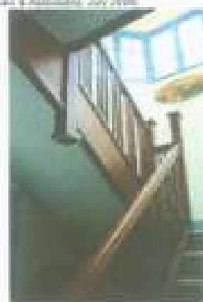
Figure 58: Cottage stairway shows typical Jefferson Jackson features including others components in this section. (Source: Graham Stokes & Associates, July 2000)
