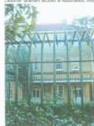
Figure 100: Sample of current security fencing arrangement (Source: Graham Brooks & Associates, July 2006)
