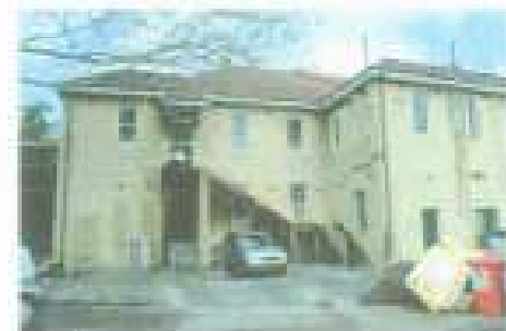
Figure 92: Two-story building at the rear of the main building. Constructed in the late 1930s. It is surrounded by extensive concrete paving. (Source: Graham Brooks & Associates, July 2006)
