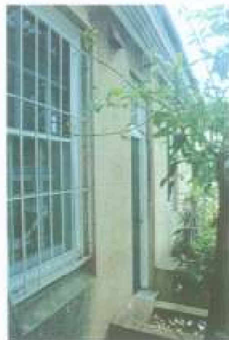
Figure 47: Lateral wall of the wing addition are retained in a superior four-pane brick. They were probably constructed in the 1930s and generally present in good order. (Source: Graham Brooks & Associates, July 2009)
