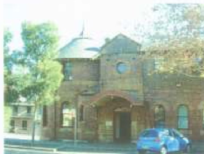
Figure 104: View of the main entrance of the former Darlinghurst Police Station showing the dark brick, face brick, sandstone and stone. (Source: Graham Brooks & Associates, July 2008)
