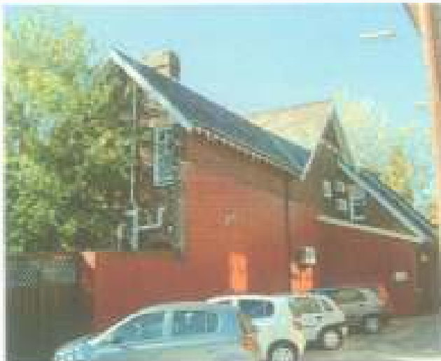
Figure 71 South side view of the Carfax Cottage presents with a 'stepped-off appearance' when compared with the land boundary. Additional storage areas were at one time situated along this building, at the red painted area where the cars are parked. (Source: Graham Brooks & Associates, July 2008)
