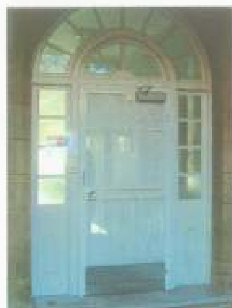
Figure 83 Original Georgian fanlight doorway, rear entrance (Source: Graham Brooks & Associates, July 2016)
