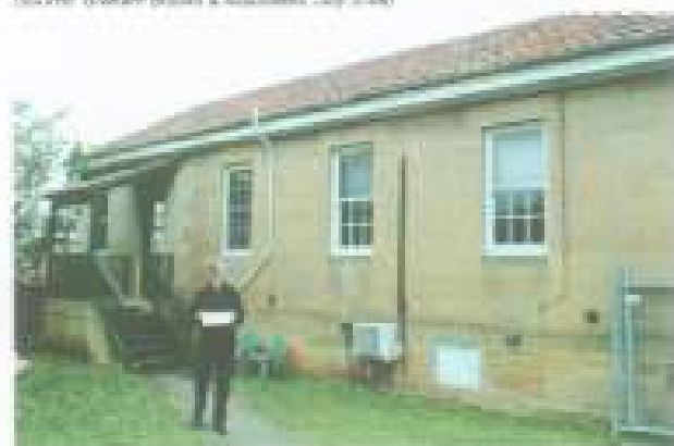
Figure 44: Ground floor wings were added in the late 1950s, being shown in the 1938 plan as a proposal. The external walls are in large part an addition. (Stucco stonework, being constructed in reinforced concrete, but with some stone elements incorporated, such as windows and lintels). While the current presentation of the buildings is highly coherent, they have been maintained in a good state of repair. (Source: Graham Brooks & Associates, July 2009)
