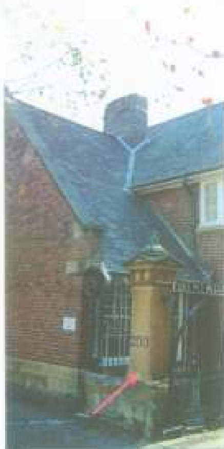
Figure 78: Example of prominent stone column with which supports the stone, face brick and iron fencing around the perimeter of the compound. The fence/wall, face brick being as a heritage item under City of Sydney Council. (Source: Graham Brooks & Associates, July 2006)
