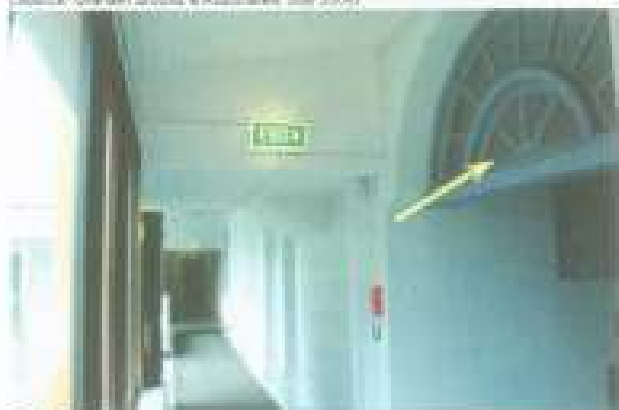
Figure 43: Passage-ways around the internal courtyard are a mixture of design and construction work. Original elements include the fanlight, the timber ceiling and the stone work. Most of the courtyard perimeter was sealed in during the reconstruction of the early 1980s. It is a mixture of aluminium framed windows and large solid style roofing. Many of the interior arrangements have been reconfigured in an ad hoc manner according to need during different eras. They thus show a consistent mixture of aesthetic preservation and sympathy with original components. (Source: Graham Brooks & Associates, July 2009)
