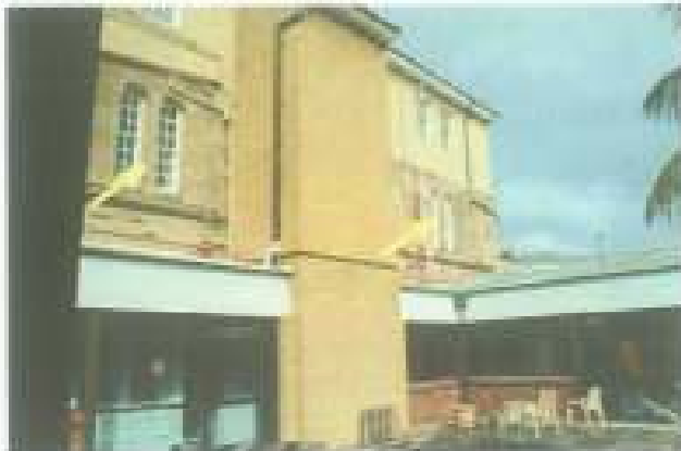
Figure 55: Interior courtyard looking towards main building. The original timber windows have been replaced at the rear and the sides of the building. The third floor was originally added in the 1930s reconstruction. The top floor windows appear to be of that era. The lower-level courtyard walkway is a mixed masonry, aluminium, glass and steel work.
