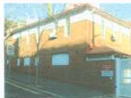
Figure 4: The Old Kitchen block at the northwest corner of the site and lying horizontally along Burton Street. (Source: Graham Brooks & Associates, July 2008)
