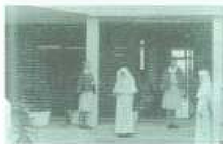
Figure 21 The newly opened 36 bed ward at the northwest corner of the site, which was completed in April 1962. (Source: St. Vincent's Archives, July 2009)
