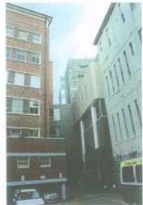
Figure 7 An image of another junction between the O'Brien Wing and the Oahli Wing, taken from Bunch Street. (Source: Graham Brooks & Associates, July 2008)
