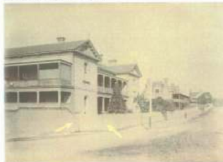
Figure 18: Photograph of the original Hospital (now the de Lacy Building), taken since 1967. It appears by the time it has been paper rendered. The view is looking south along Victoria Street towards Police Street. The stone pillar boundary markers are clearly seen at the corner of the property. The next building visible up the hill is the Sisters of Mercy Convent. (Source: St. Vincent's Hospital Archives, July 2008)
