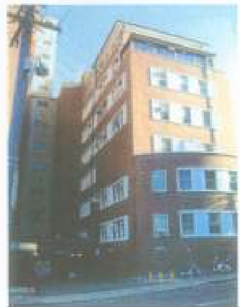
Figure 6 The image above shows the junction between the O'Brien Wing and the Oahli Wing to the west (left), with emergency vehicle access under the junction. (Source: Graham Brooks & Associates, July 2008)
