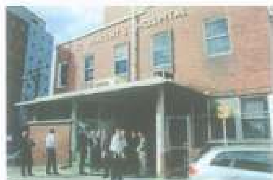
Figure 2 The new glass entrance way to the O'Brien Wing, which presents a relatively poor view of repeat, and widens some of the acoustic necessary for contemporary use, such as for air-conditioning units. (Source: Graham Brooks & Associates, July 2006)
