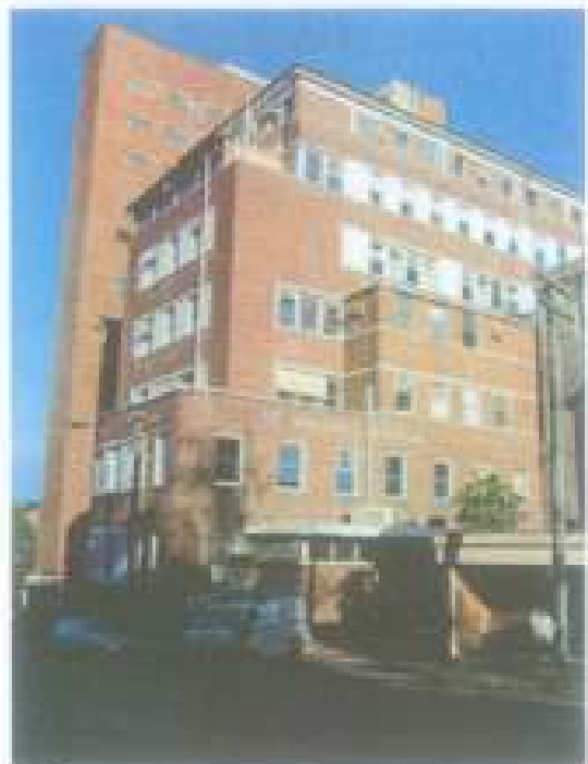
Figure 1 The O'Brien Wing from Burton Street looking east. The building is in the modern style of the late 1930s, characterised by clean horizontal delineations. (Source: Graham Brooks & Associates, July 2006)
