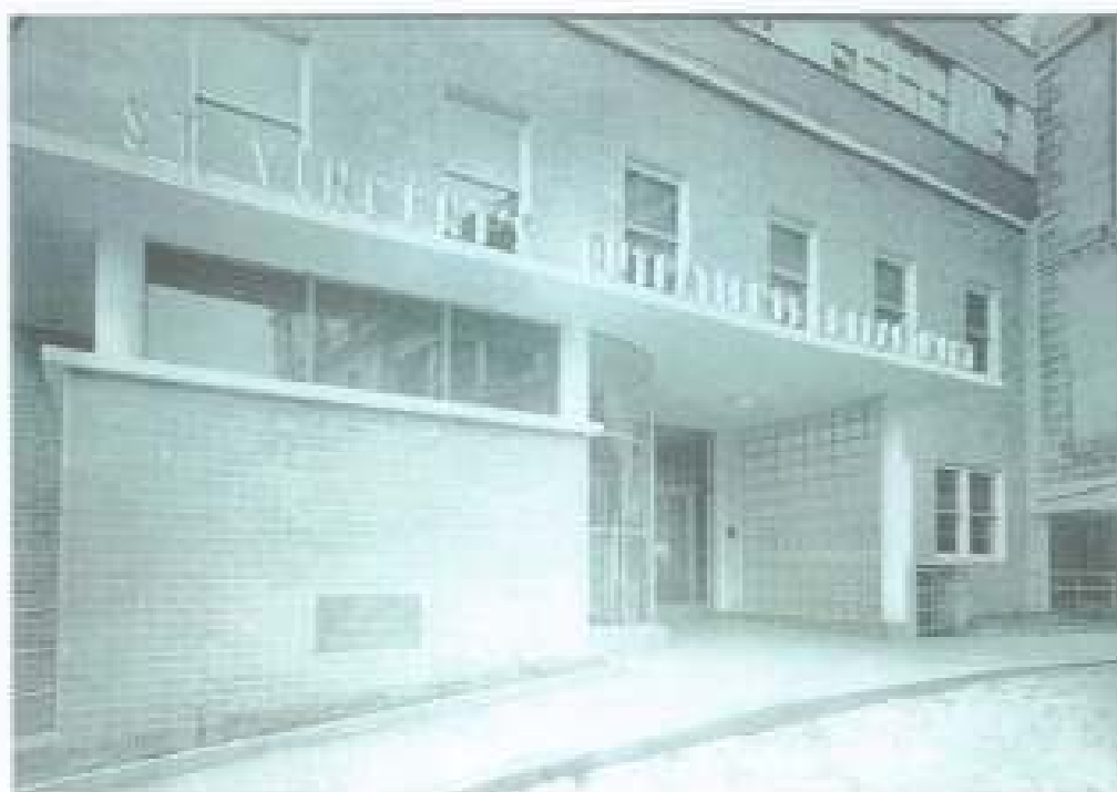
Figure 10 Photograph taken January 1941 of the entrance to the new building, which, as noted above is an Outpatients Block. The new building presents as state of the art, in the then new modernist style. (Source: St. Vincent's Archives, July 2006)
