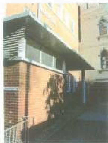
Figure 27 An image of the side area of the subject building where the street wall (Barton Street) and showing the close proximity of the subject building to the old Lane Building. It also indicates the generally good state of repair of the face brick and concrete work. (Source: Graham Brooks & Associates, July 2008)
