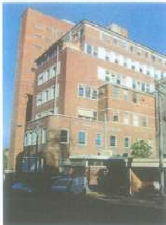
Figure 28: View of the southwest corner of the building taken from Sullivan Street. This image illustrates the nature and the proportions for the architectural units. (Source: Graham Brooks & Associates, July 2008)
