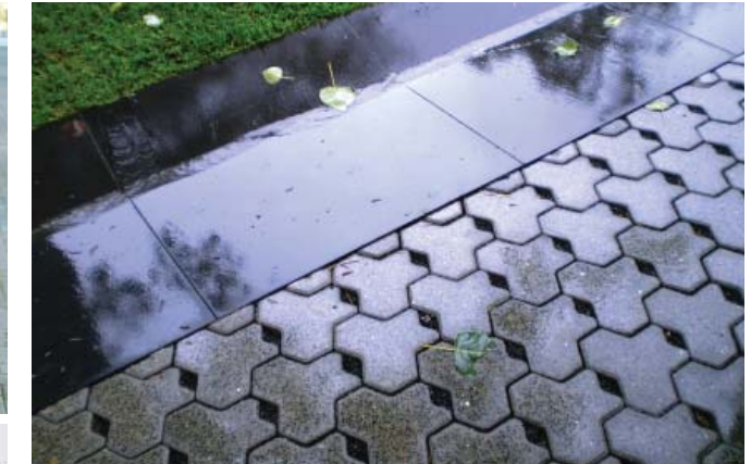
Above: Permeable pavements minimise impervious areas and allow for stormwater infiltration.
